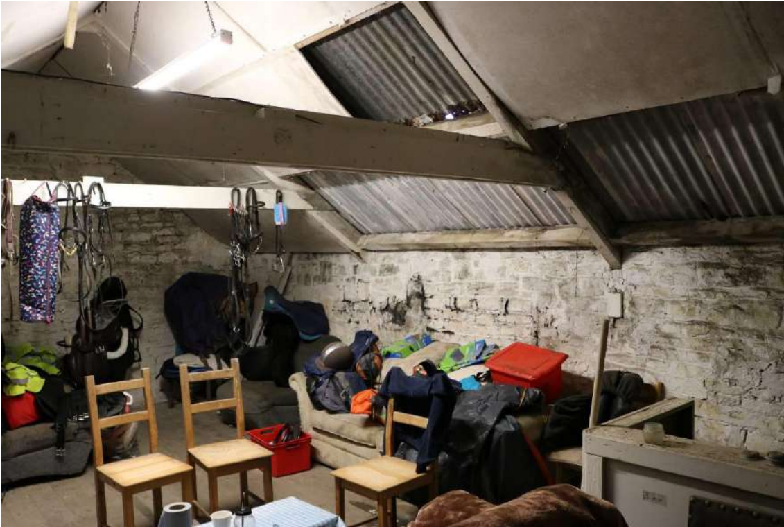
Image EDP 11: View of the first floor space at the west end of Structure A.
