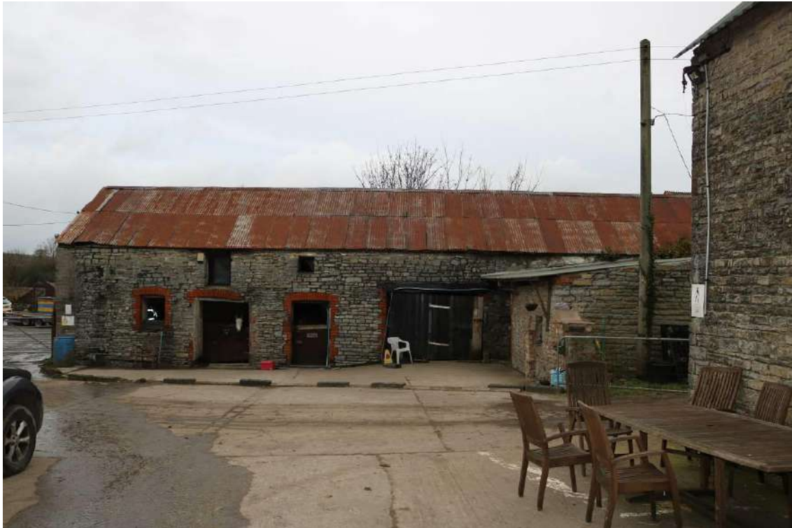
Image EDP 5: View of the south-facing elevation of Structure A from within the farmyard and here showing the stratigraphic relationship between the two early phases. The earliest element of the building can be discerned where the double doors are visible.
