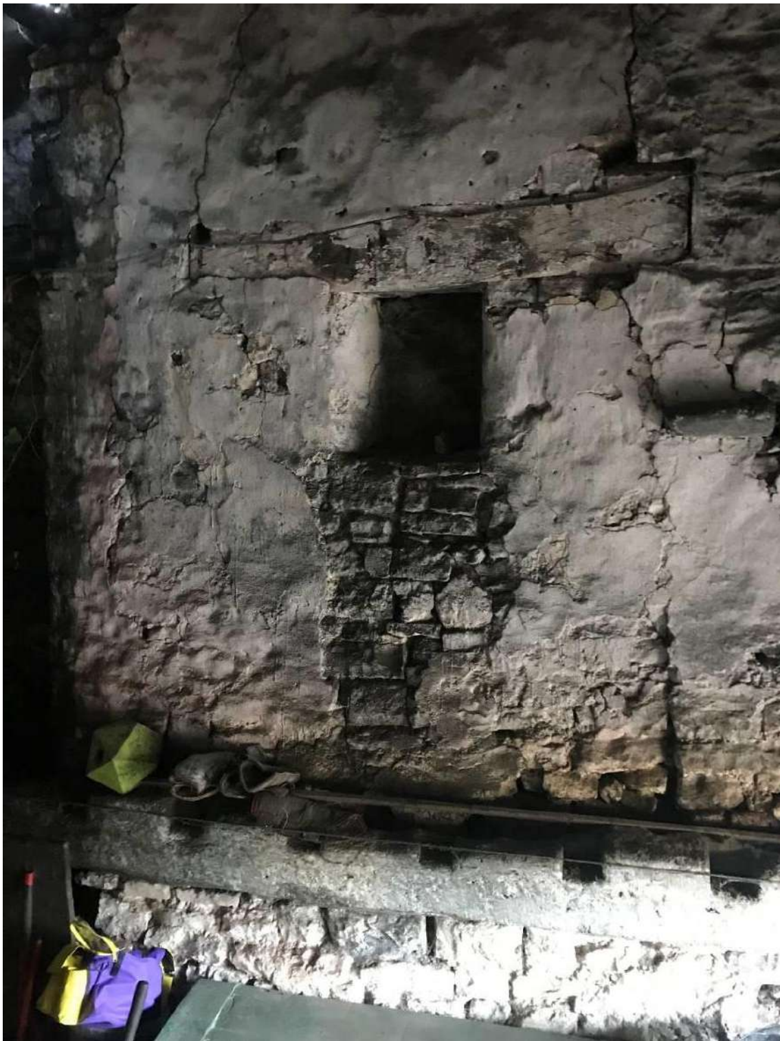
Image EDP 7: View of the east-facing gable of the earliest phase of Structure A, here illustrating the infilled window opening and the timber beam.
