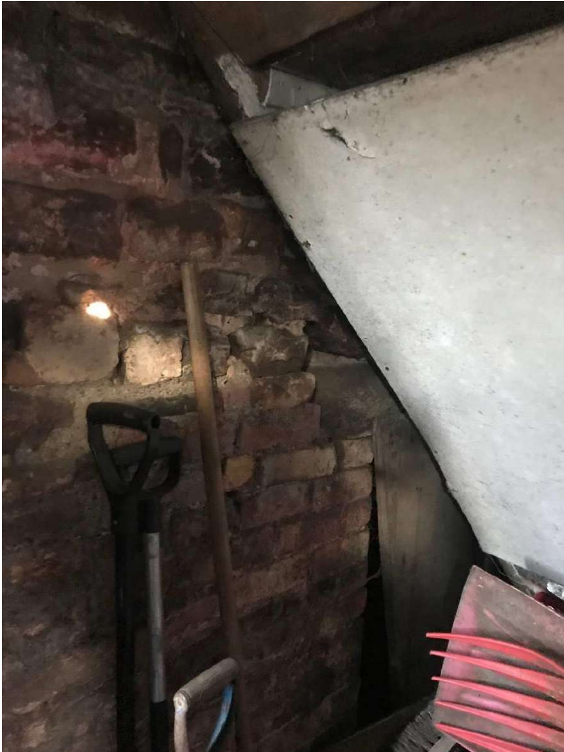
Image EDP 9: View of the fireplace concealed by the modern timber staircase on the west side of the earliest section of Structure A.
