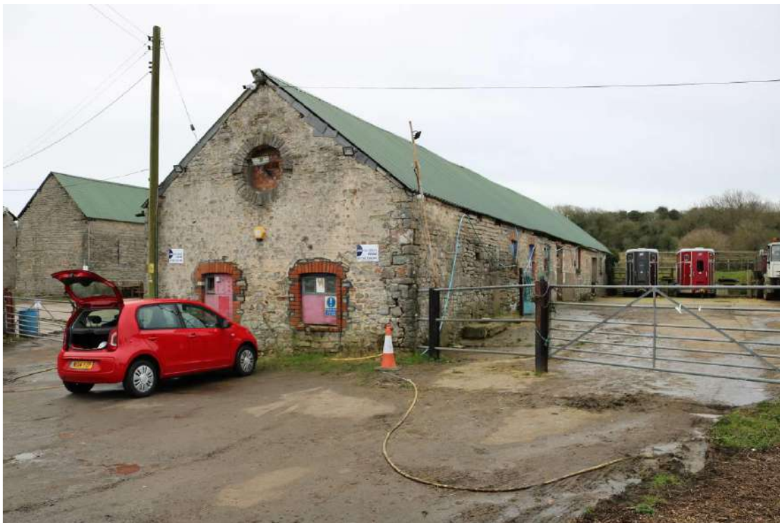
Image EDP 4: View of Structure C looking south from the old course of Lavernock Road and showing the similarity in the form of the window openings with Structure A further east.
