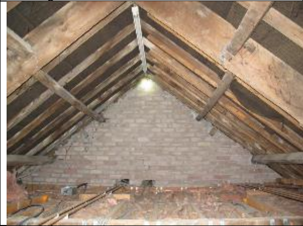
Building 1 loft void interior
