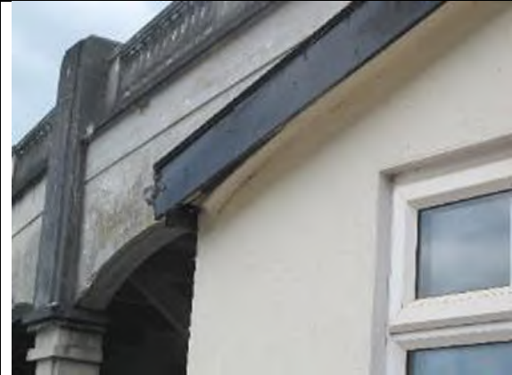
Building 6 – external features
