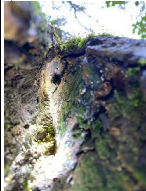
Tree 20 Interior of wound feature
