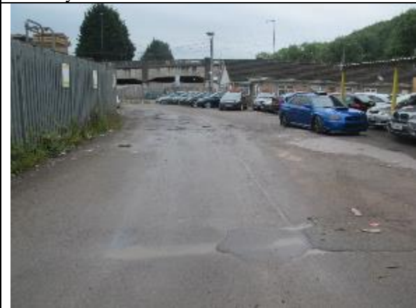
Area of hardstanding to the north of the site
