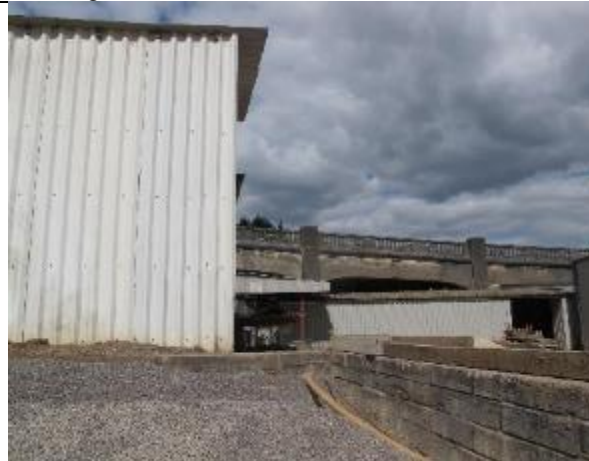
Building 6 and viaduct
