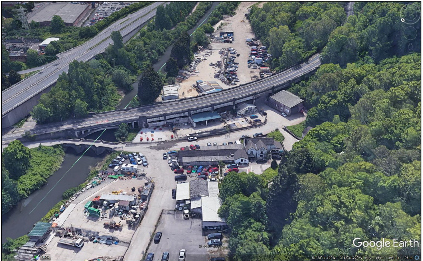
Figure 9.2: Google Earth view looking downstream at Existing Bridge
