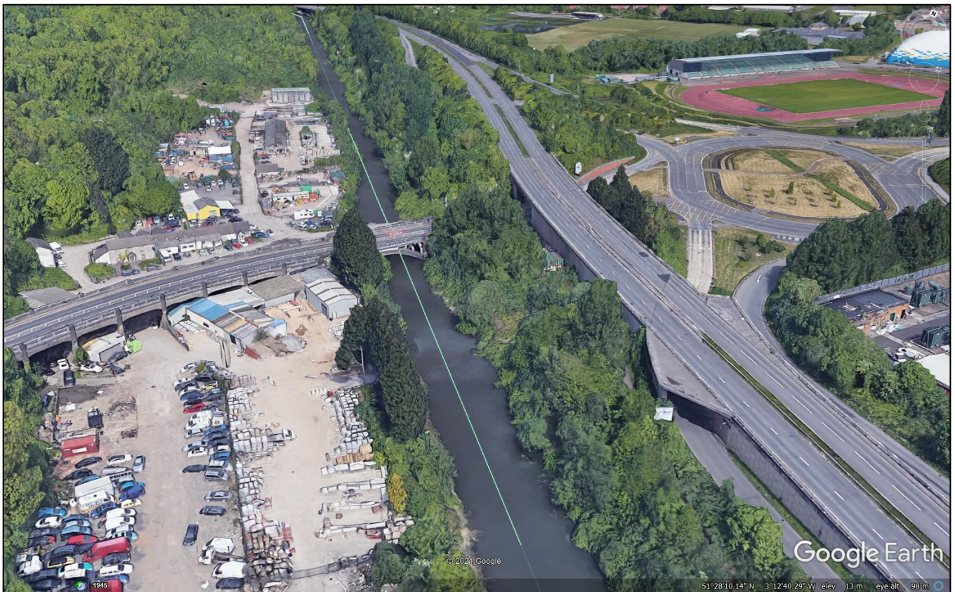
Figure 9.1: Google Earth view looking upstream at Existing Bridge
