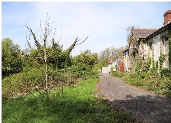
3: View northwards along main façade to service block
