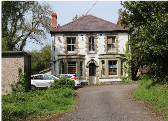
1: View northwards along main drive
