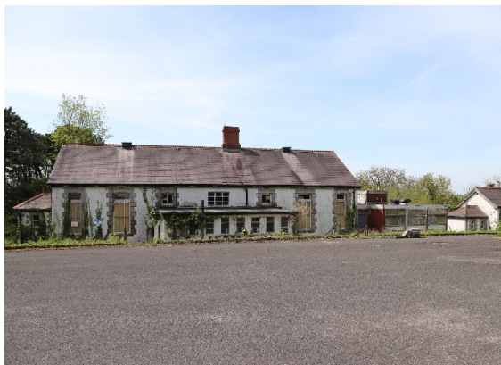
2: Service block (left) with later addition and wards (right)
