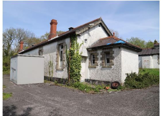
4: Western façade of wards (left) with mortuary to rear
