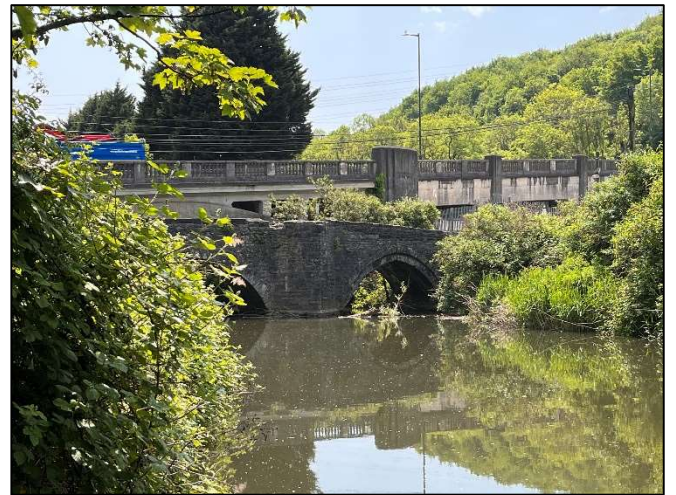
Existing Leckwith Quay Bridge to remain
