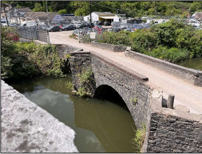
Existing Leckwith Quay Bridge to remain
