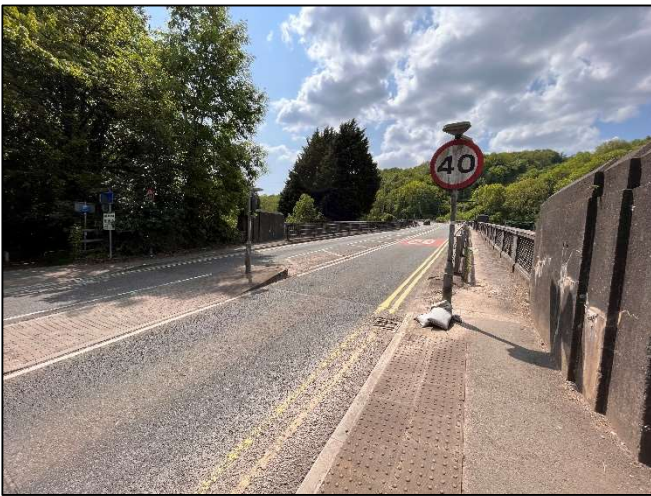
Leckwith Road / Leckwith Bridge
