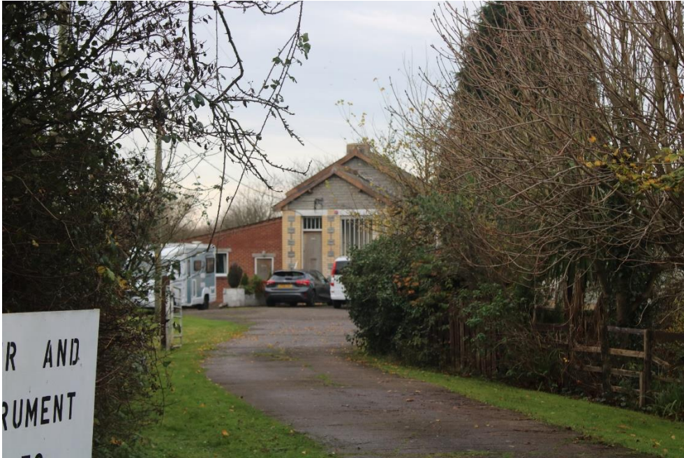
Photo 21: View west from Fort Road of the former Lavernock Station buildings
