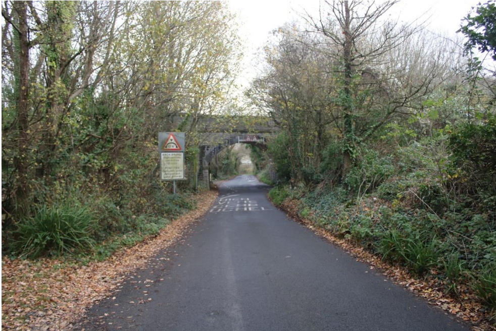
Photo 23: View north along Fort Road to the railway bridge
