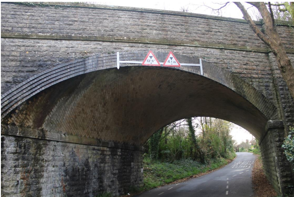
Photo 24: View south of skewed brick arch of railway bridge over Fort Road
