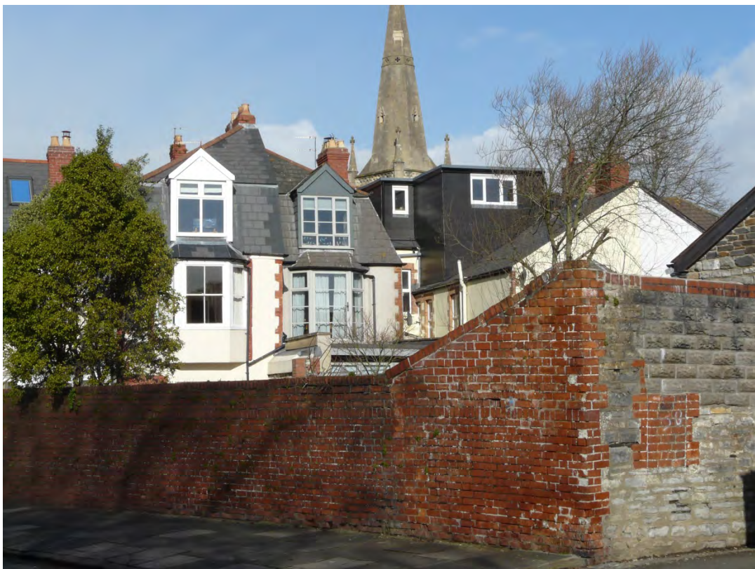
Photo 2: View of the rear dormer additions from Grove Terrace
