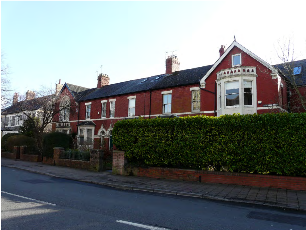
Photo 1: View of roof lights on the front elevation of the appeal property and context of street scene
