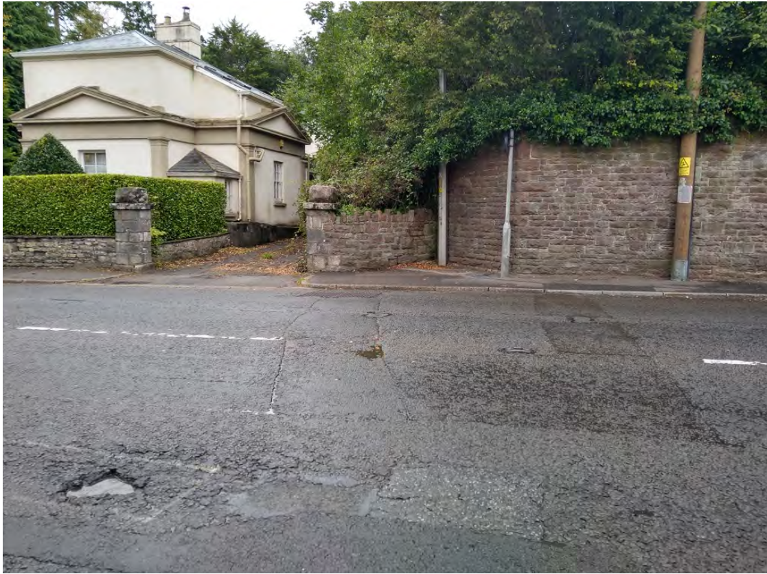
Figure 2 Existing Bolston House Access
