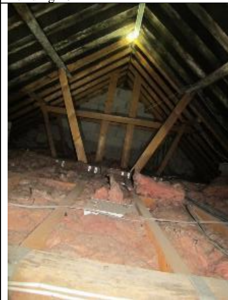
Building 1 loft void interior
