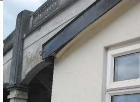
Building 6 – external features
