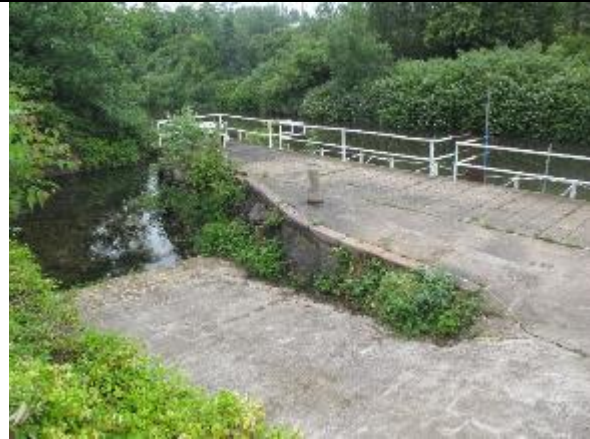
Jetty to the east of the site
