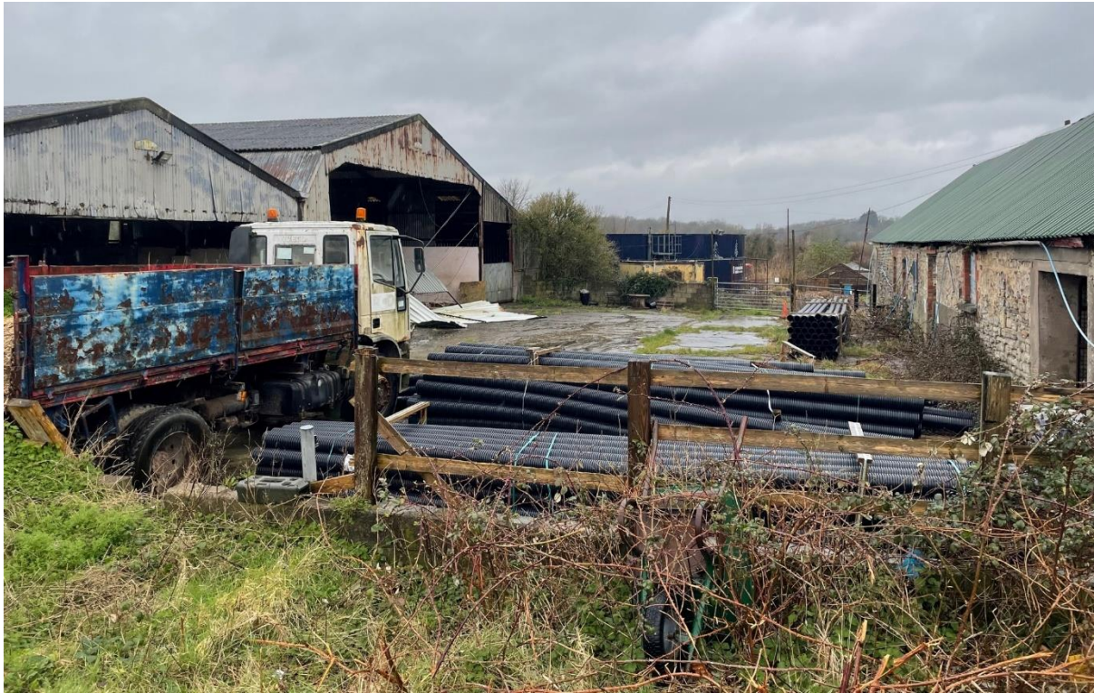
Plate 12.21: View looking north west from the south-west corner of Lower Cosmeston Farm and illustrating the relationship between the historic farm buildings on the right-hand side and the mid-20 th century and later agricultural structures that have been added on the left hand side.
