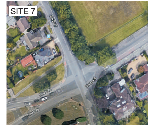
Lavernock Rd/Dinas Rd/Victoria Rd Cross Roads
