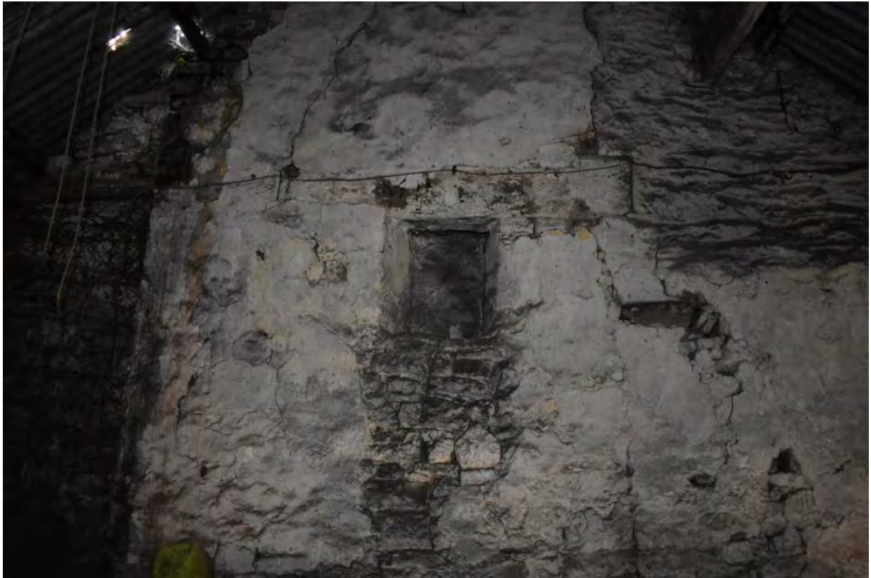
(Figure 6. View of blocked-up window within the east wall )
