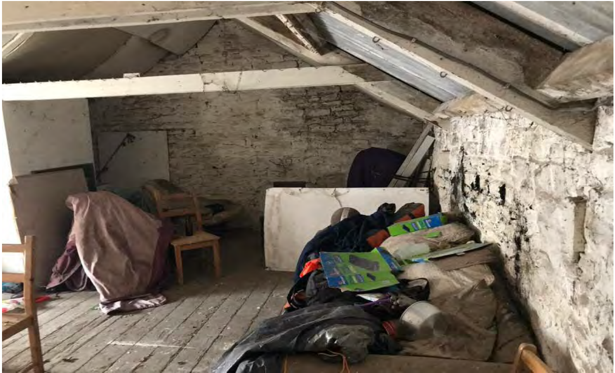
(Figure 7. View of the upper level of Lower Cosmeston farmhouse)
