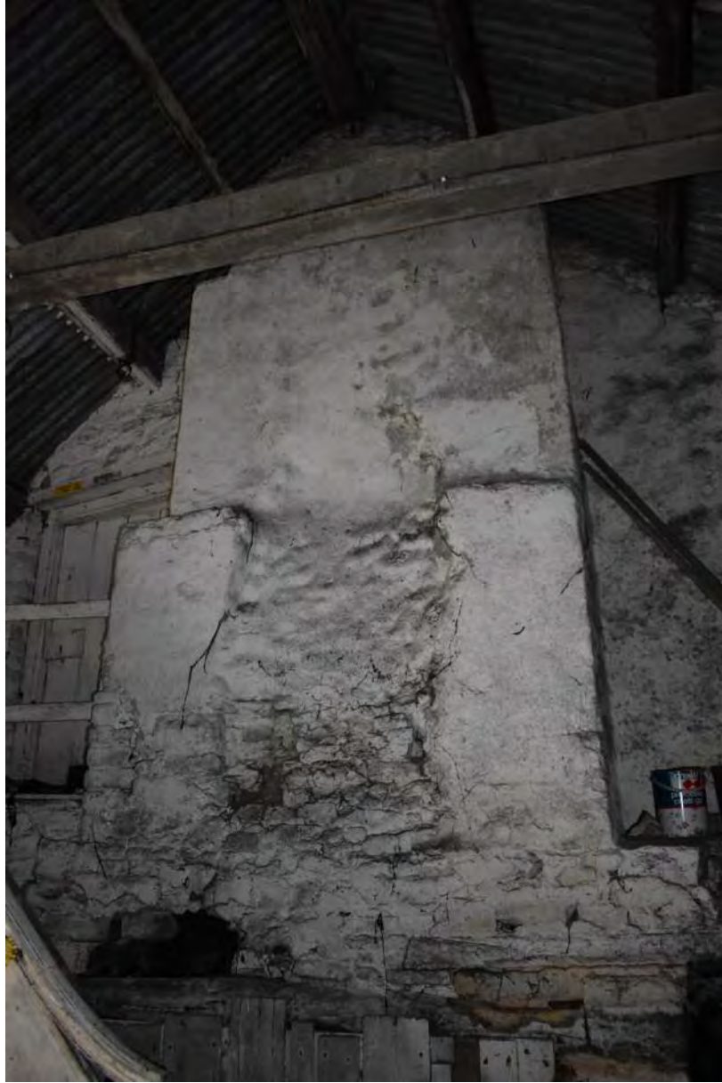
(Figure 5. View of the internal chimney stack. The external stairs are to the left of the stack )
