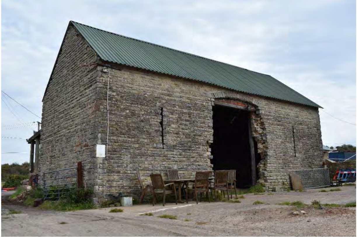
(Figure 10. View of the threshing barn from its east angle )
