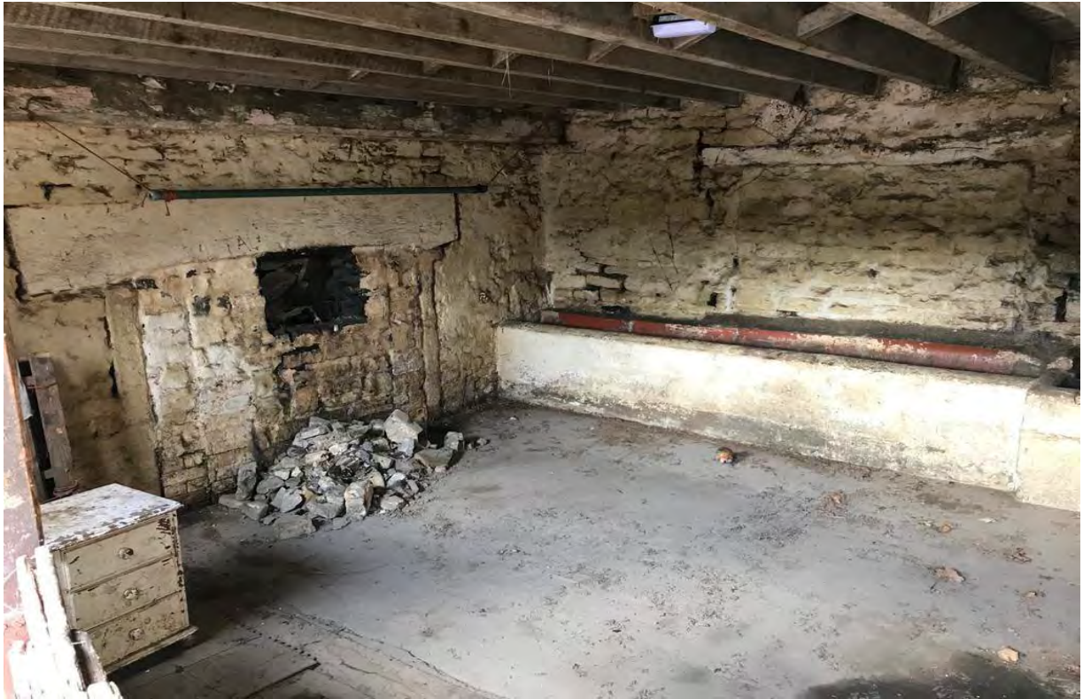
(Figure 3. View of the parlour area showing the fireplace and wooden corbel. The staircase is just out of view to the left)
