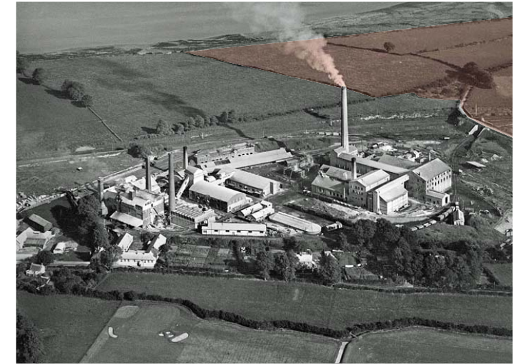
Cement works looking east
