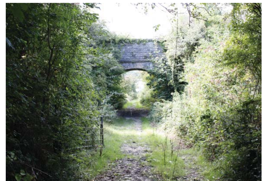
Arched bridge, site photo
