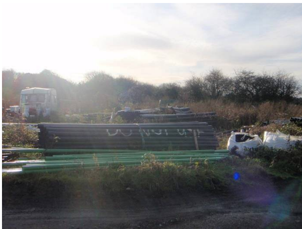
Plate 15: Storage area – pipes and asphalt
