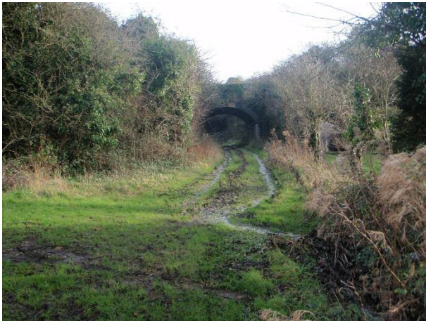
Plate 9: Historical railway line and bridge
