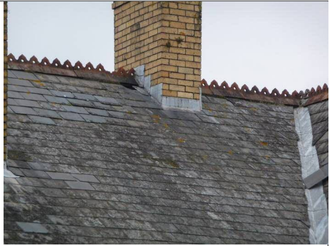
Photo 18: Roof of Building 1 showing missing tile.
