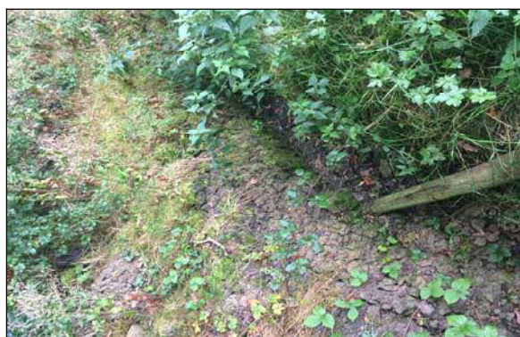
Figure 13: Dry ditch TN12
