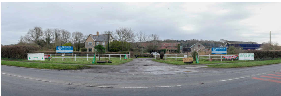
Image EDP 1: View and appearance of existing buildings within the area of Green Wedge in question, from the access off the B4267.
