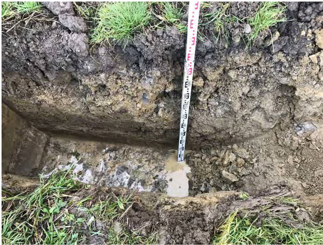
TP114 – Longwall Face C
