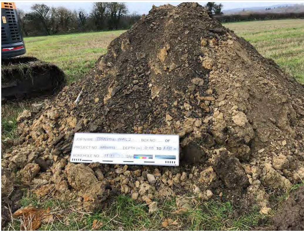
TP111 – Spoil Pile
