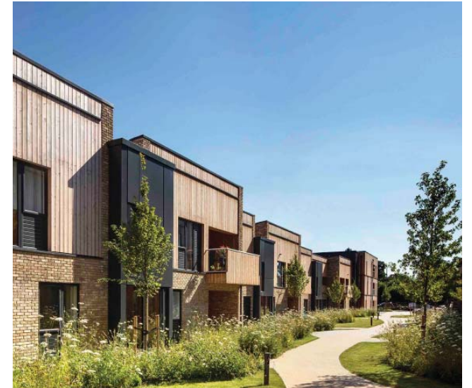
Clock House Gardens, Welwyn Garden City, Stockwool
