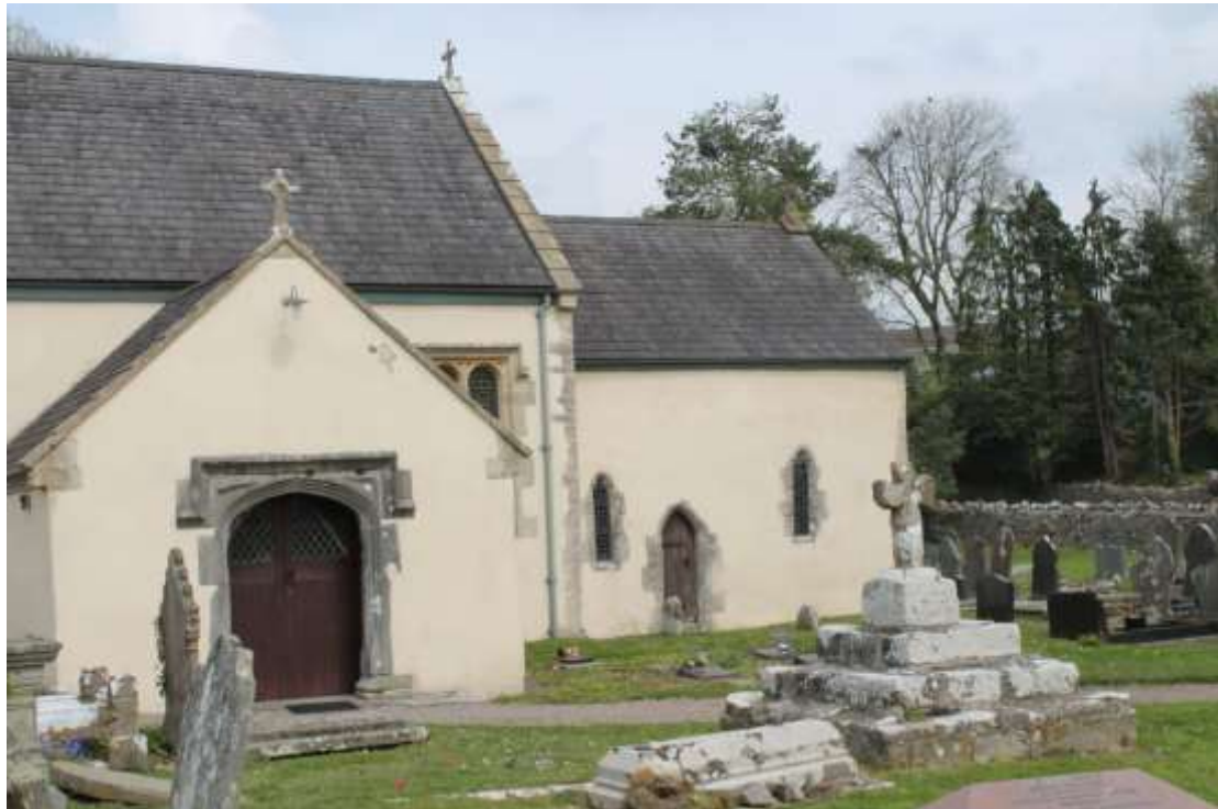
Photo 2: Colwinston church cross and church viewed from the south
