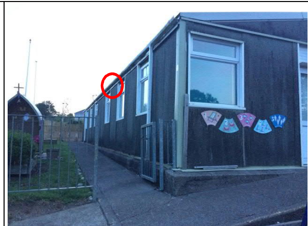
Photograph 2: Building 2 - west face. Roost re-entry on 02/08/2019 location circled.
