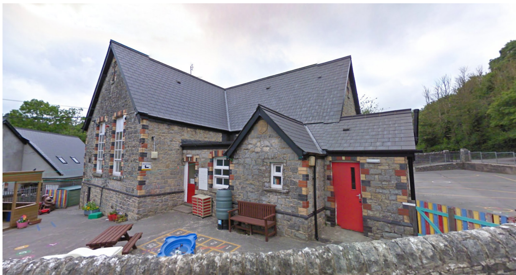
Right: Llancarfan Primary School - existing school buildings and external areas
