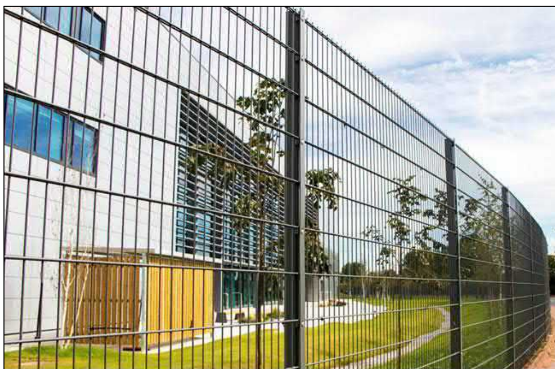
Figure 3-1: Fence Boundary Construction
