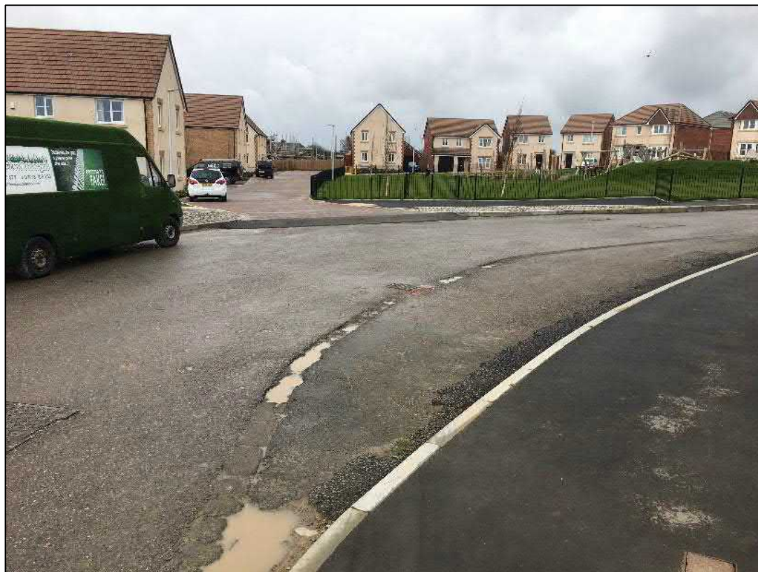
Figure 2-4: Localised Carriageway Widening on Rhoose Way
