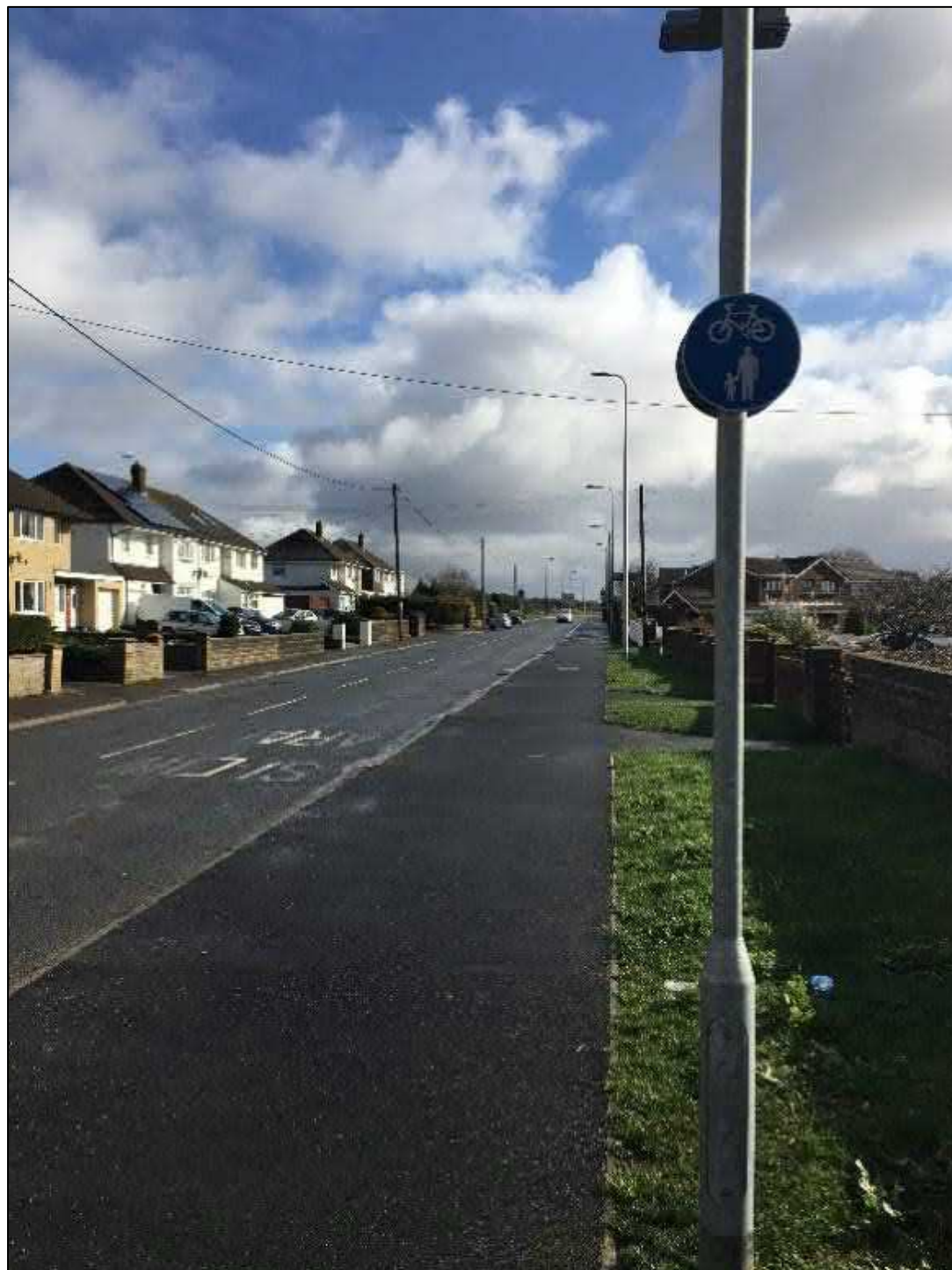
Figure 2-11: Porthkerry Road Shared Footway / Cycleway
