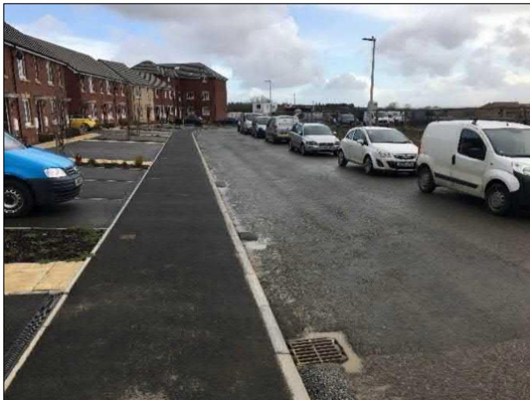
Figure 6-2: On-Street Parking along Rhoose Way
