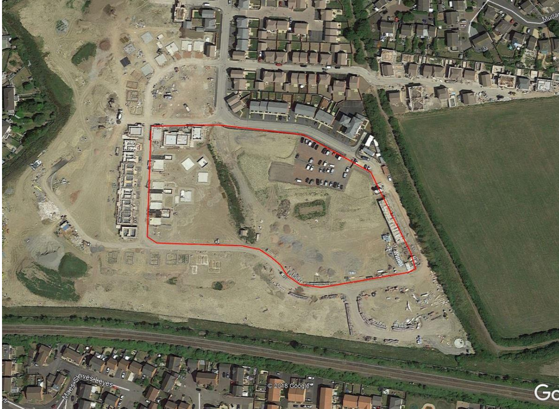
Figure 2: Aerial image of the site area from Google maps with the school site area overlaid in red (image supplied by AECOM)
