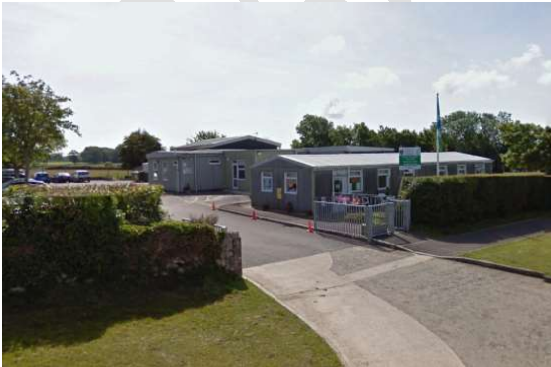
Photo 3: View southeast from the road across the school buildings and northern car parking area
