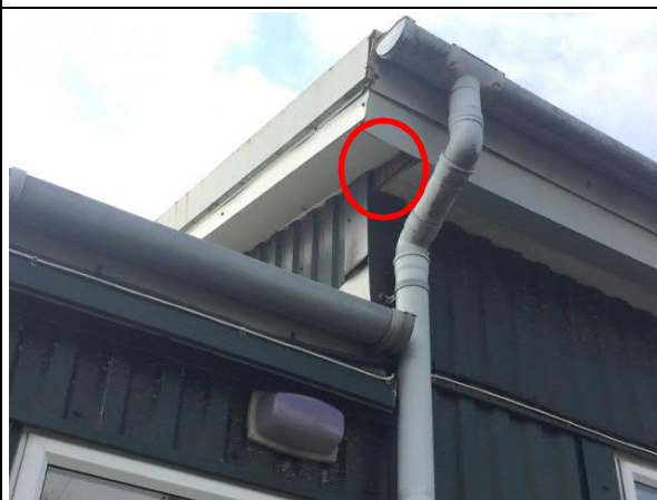
Photograph 5: Building 1. Potential roost features - Gap between soffit. Not roosting activity recorded.
