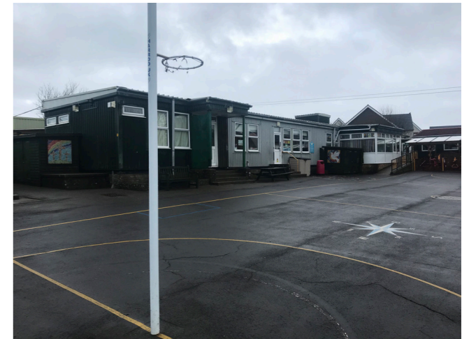
Existing school buildings at the northern end of the site.
