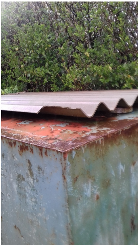
Plate 26: Cement asbestos roof sheet, located in Model Farm.
