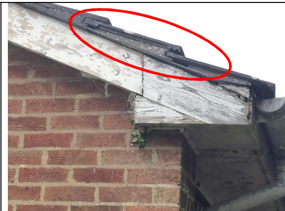
Photograph 2: Building 2, north-east corner.
