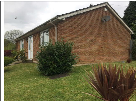
Photograph 1: Building 2, east and south faces.
