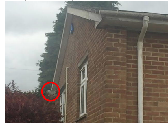
Photograph 3: Building 2, west face.
