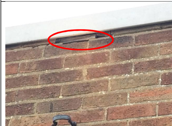
Photograph 49: Building 12, a close up of the feature identified in Photograph 48.
