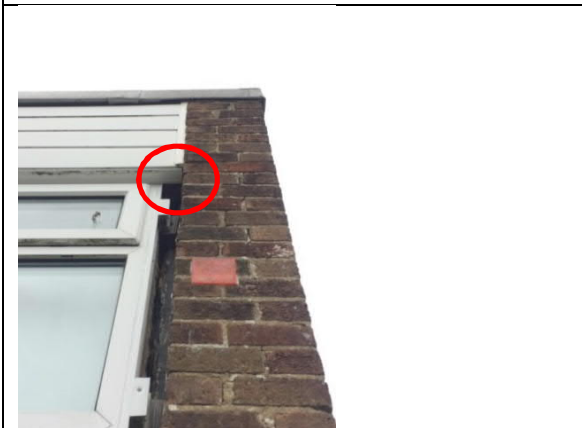
Photograph 47: Building 12, the south-east corner.
