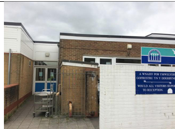
Photograph 50: The east faces of Building 13.
