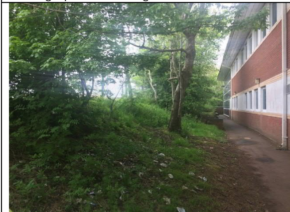
Photograph 31: Building 6, the north face and dense scrub with row of trees.
