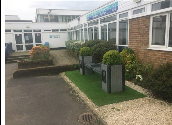
Photograph 28: Building 9 and Building 4.
