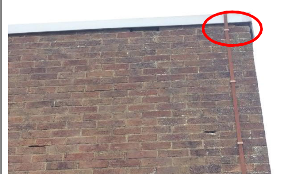
Photograph 42: Building 10. The south-west corner.
