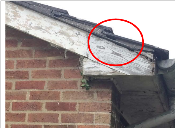
Photograph 25: Building 2, the north-east corner.
