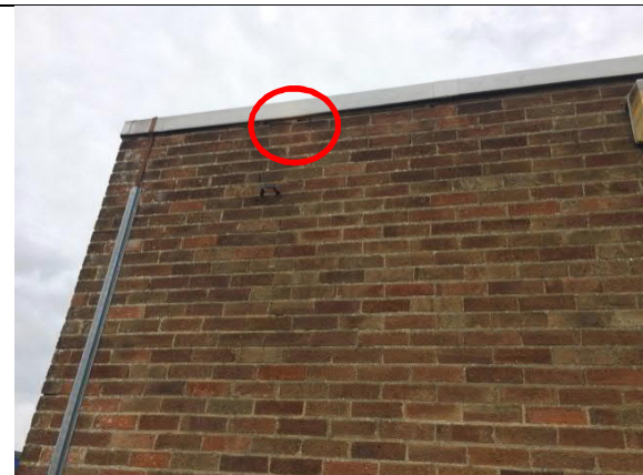
Photograph 48: Building 12, the east face.
