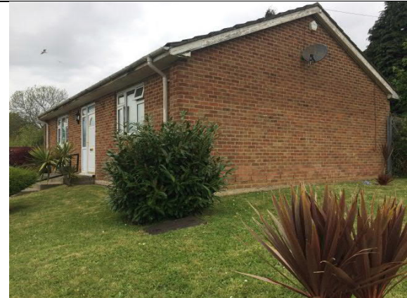
Photograph 24: Building 2, the east and south faces.
