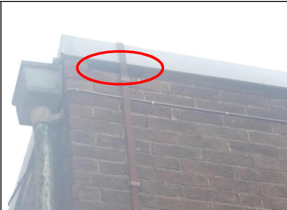
Photograph 40: Building 10. The north-west corner.
