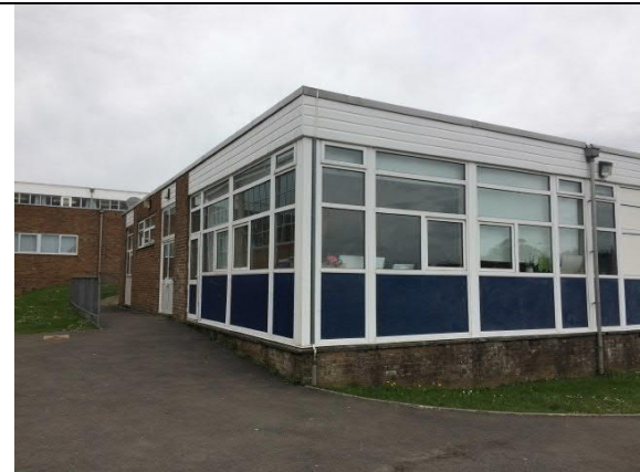
Photograph 46: Building 12, the south and west faces.
