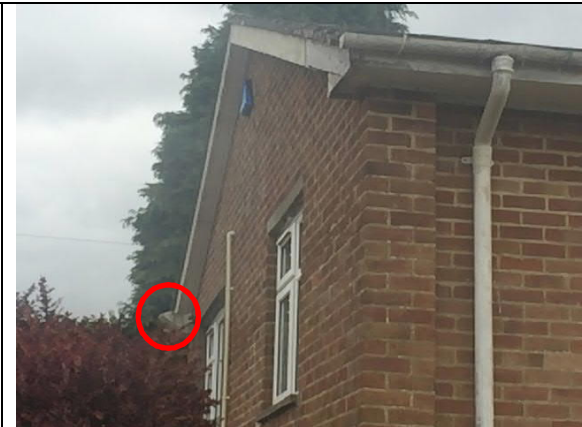
Photograph 26: Building 2, the west face.
