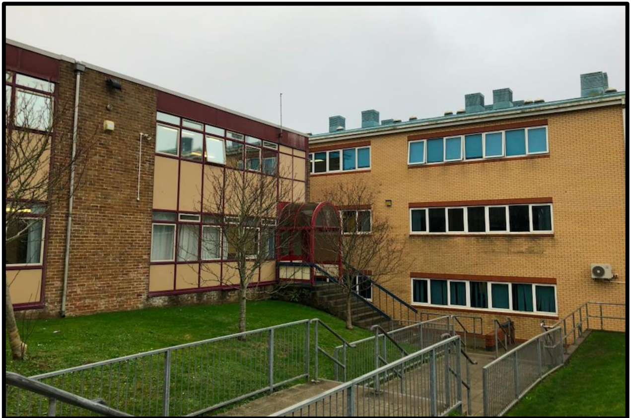
Figure 2 – Buildings on the west part of the school
