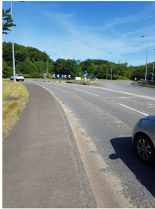
Photograph 3: A4050 Port Road Roundabout
