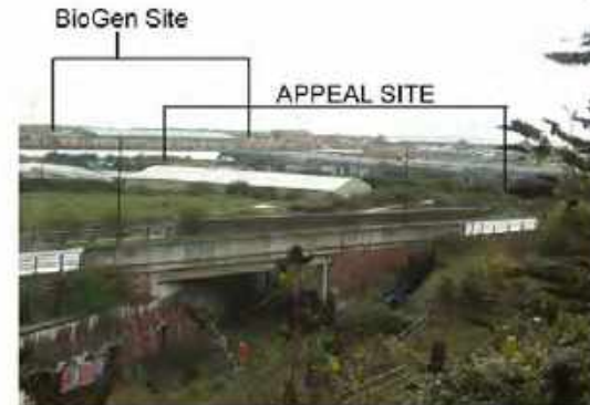
Photograph 7, View from Dock View Road, Lower Pyke Street Junction
