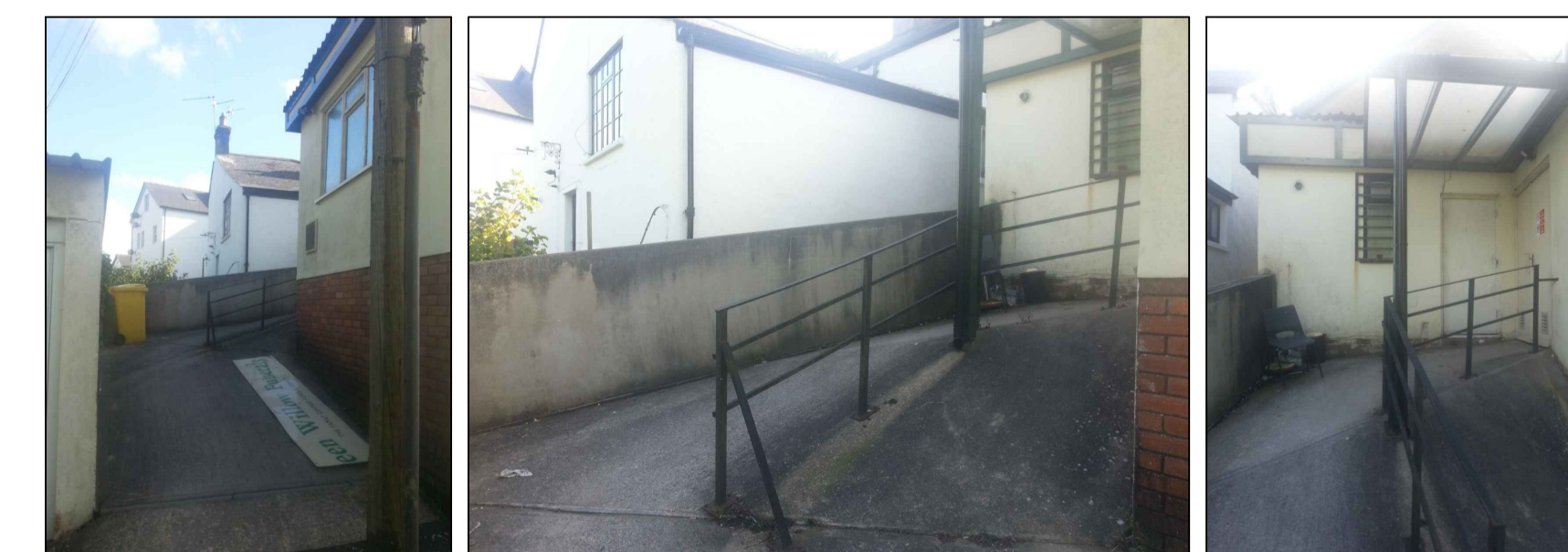
PHOTOS SHOWING EXISTING RAMP & WALL TO BE REMOVED.
