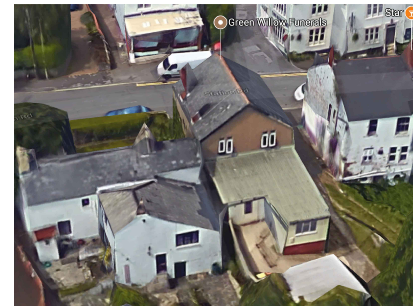
VIEW ON REAR OF PROPERTY
