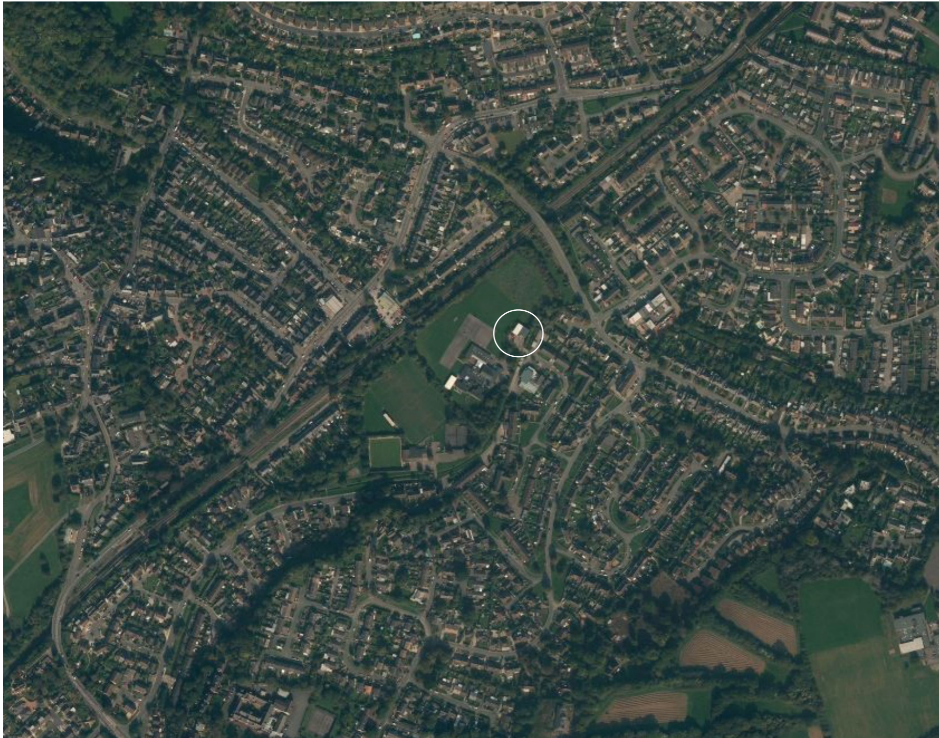
▲ AERIAL IMAGE OF DINAS POWYS COMMUNITY LIBRARY, SHOWING THE SITE WITHIN THE CONTEXT OF THE SURROUNDING AREA N
