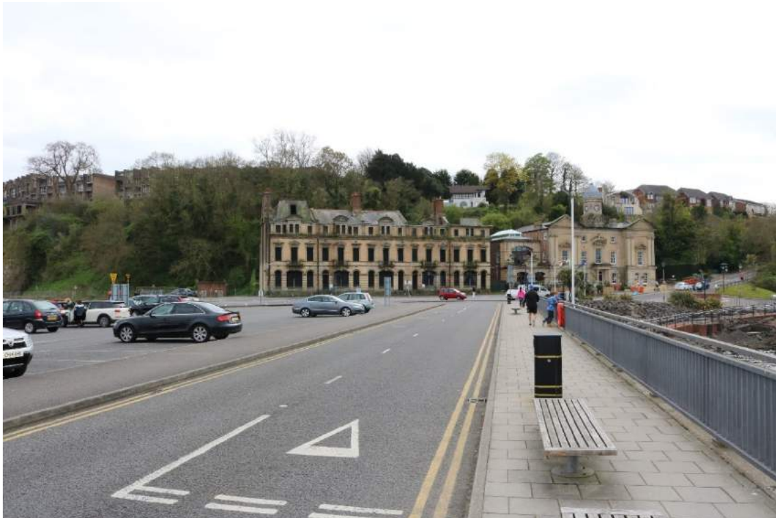
Image EDP 18: Close-up of the Custom House and Marine Buildings from the southern end of the Barrage, showing the proposed development site behind.
