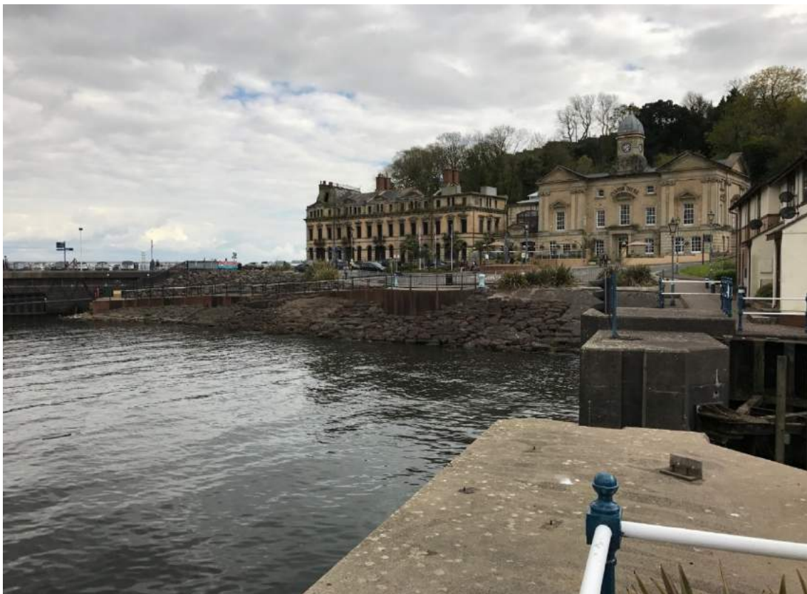
Image EDP 19: View of the Custom House and the adjacent Marine Buildings (now derelict) from the east end of Penarth Marina, here highlighting the historical functional relationship between the two, which endures despite the redevelopment of the surrounding spaces in the late 20th century.
