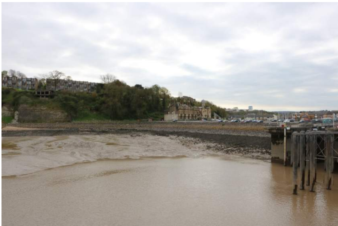
Image EDP 9: View looking south west from the outer basin at the entrance to Cardiff Bay, here showing the screening effect of the natural topography concealing the tower of St. Augustine's Parish Church.
