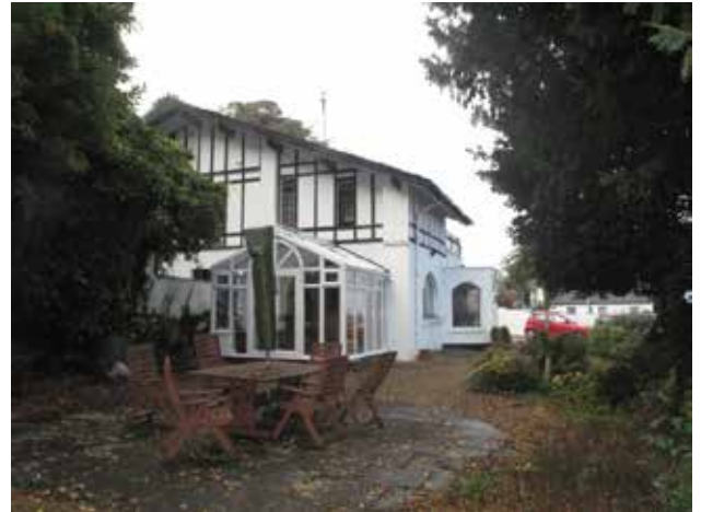
View of eastern elevation Northcliffe Lodge
