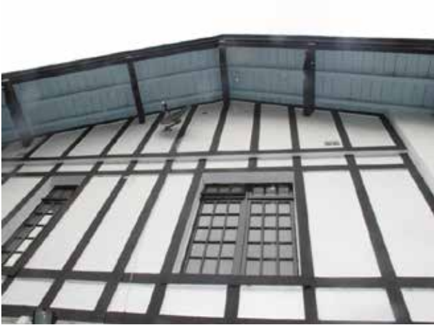
View of close fitting extended eaves
