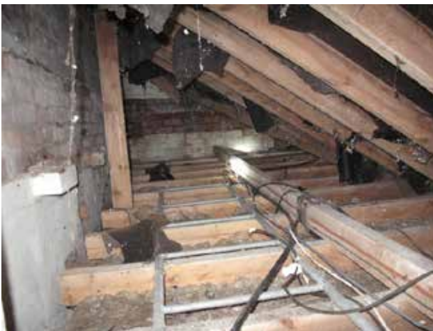
Attic void above outbuilding
