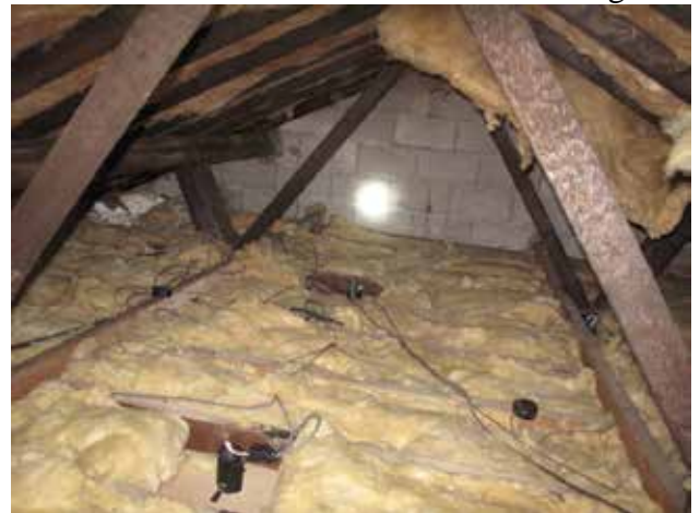
Attic void above extension
