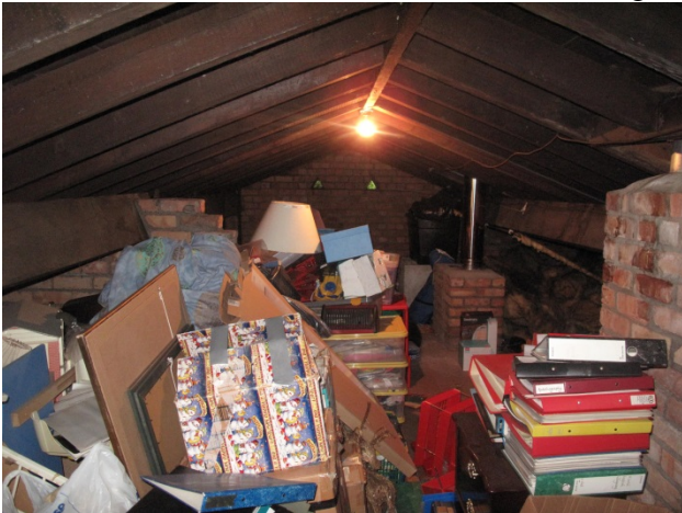
Attic void in main house
