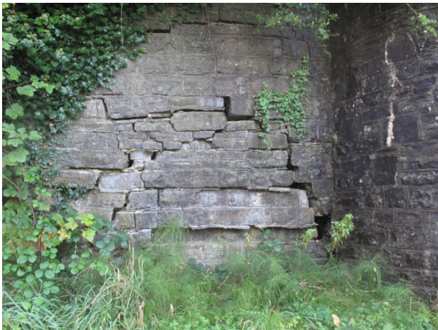
Cracks in retaining wall
