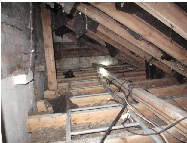
Attic void above outbuilding
