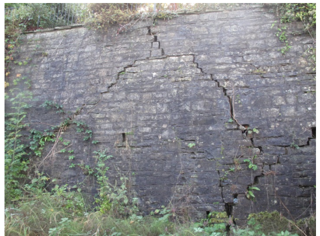
Cracks in retaining wall
