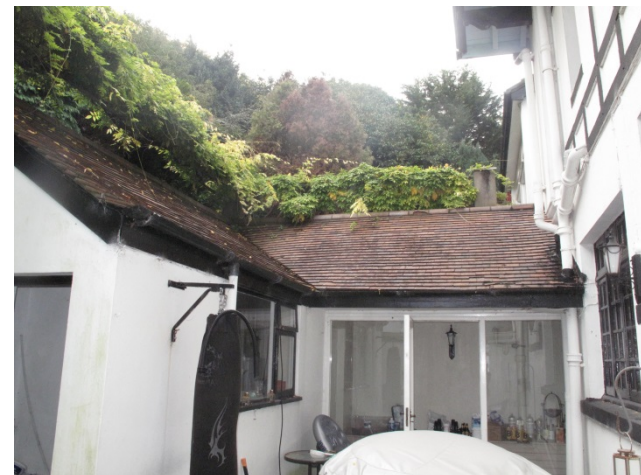
View of outbuilding
