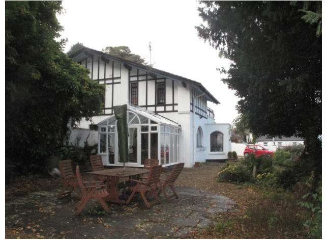
View of eastern elevation Northcliffe Lodge
