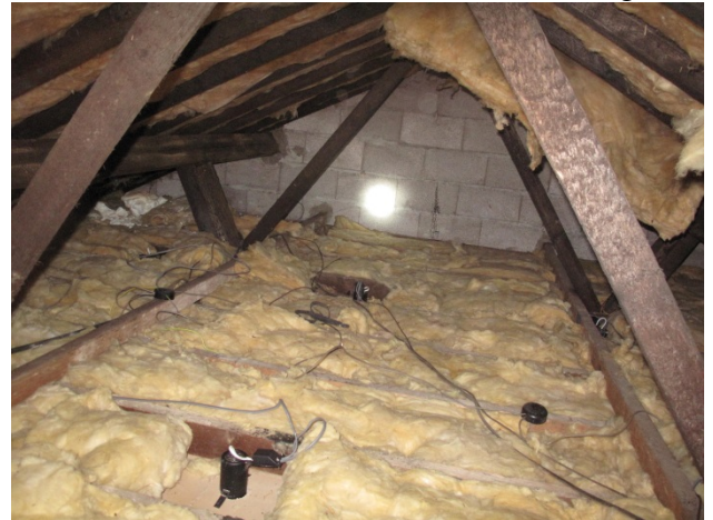
Attic void above extension
