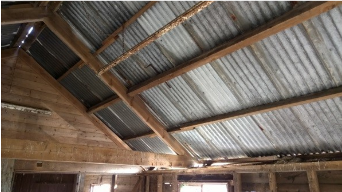
Figure 4 – Internal View of Roof
