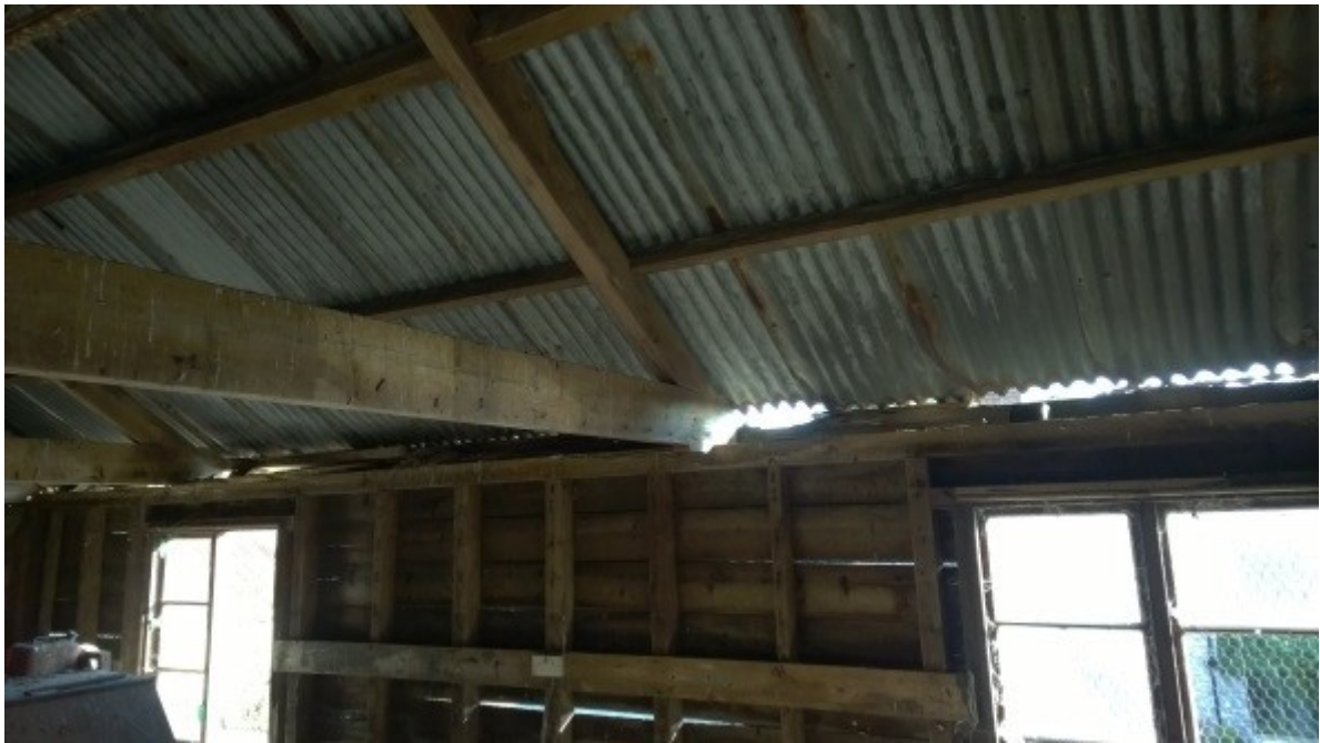
Figure 7 – Openings in External Fabric
