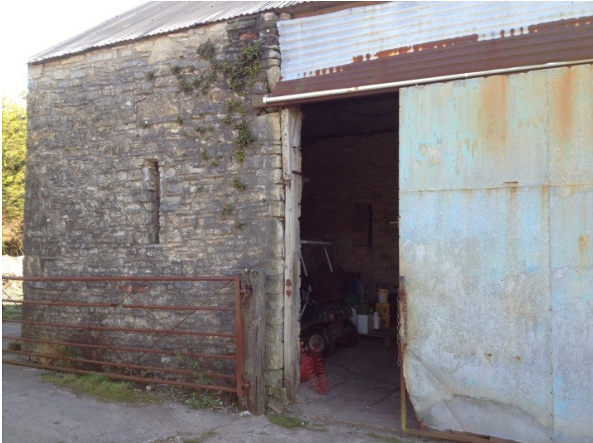
Figure 9 – External View of Barn
