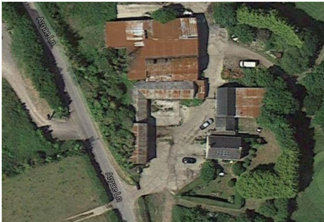
Figure 1 – View of Existing Site
