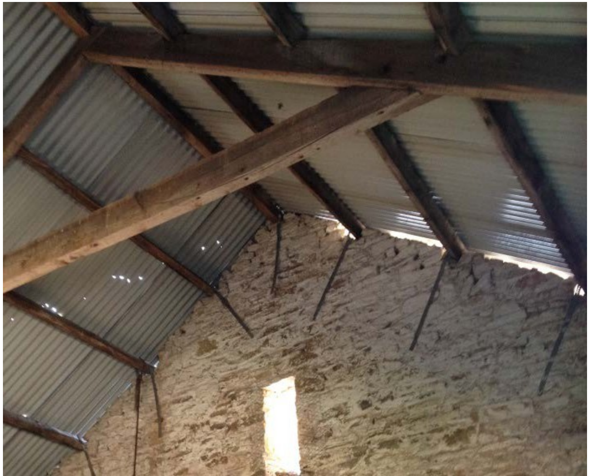
Figure 10 – Roof of Stone Barn
