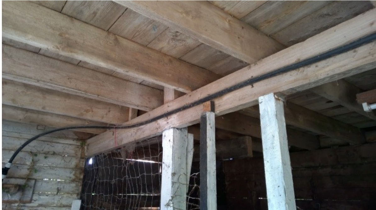
Figure 6 – Floor Joist Beam Junction
