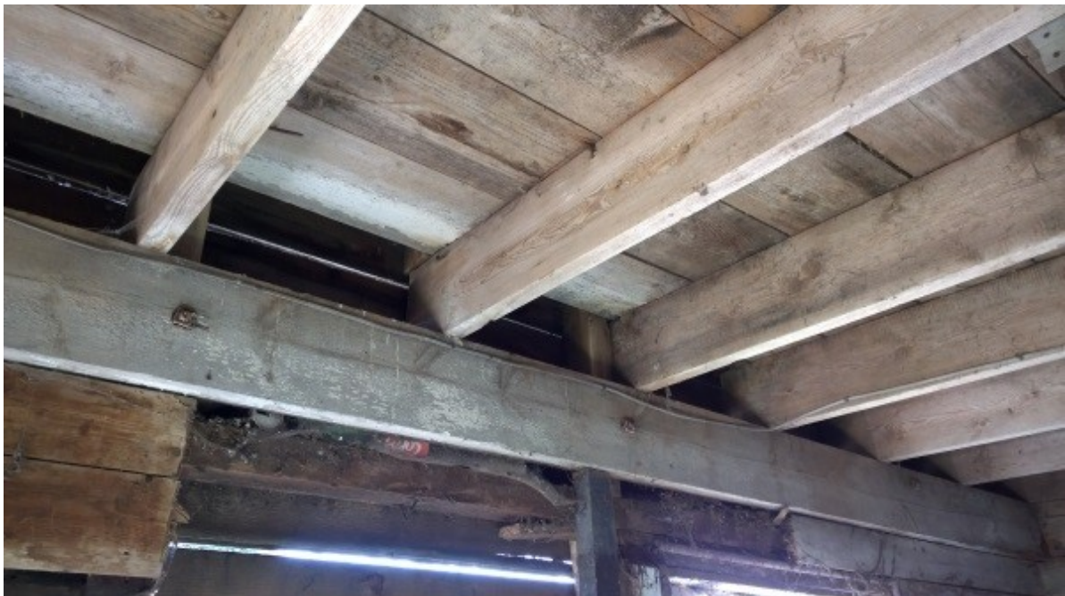
Figure 5 – Floor Joist Junction at External Wall
