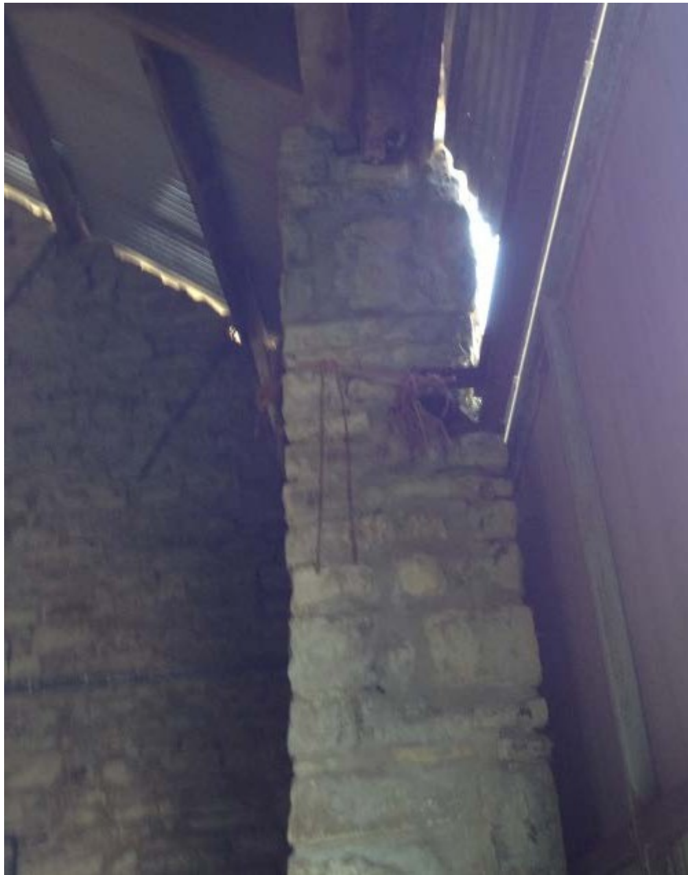
Figure 11 – Stone Barn External Wall
