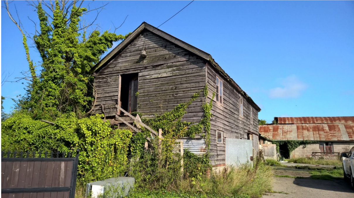
Photo 1: Double storey timber barn
