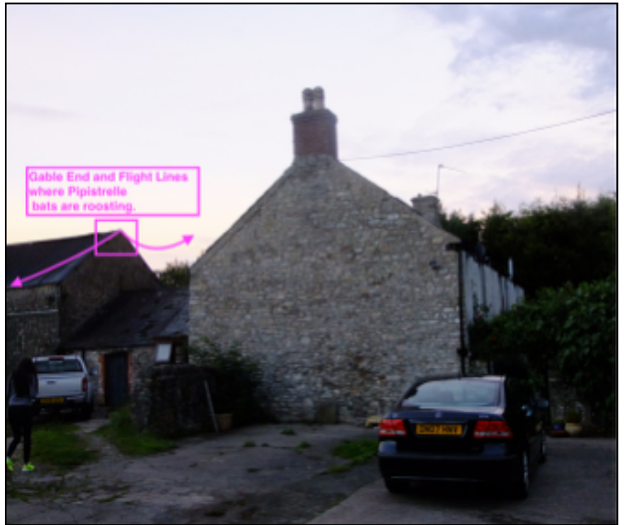
Common Pipistrelle exit point out of stone barn
