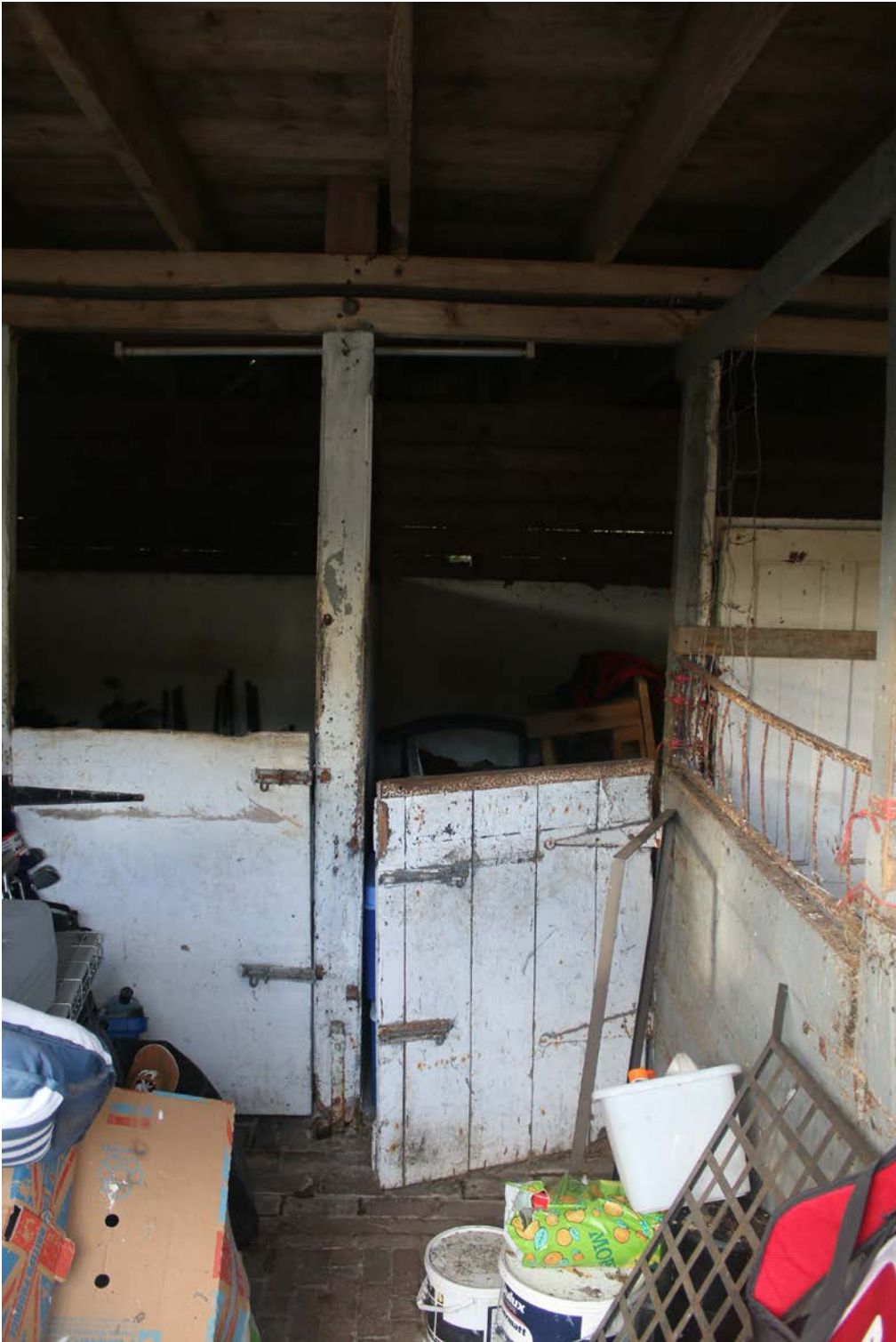
Image EDP 10: Representative photograph showing the interior of the stable block
