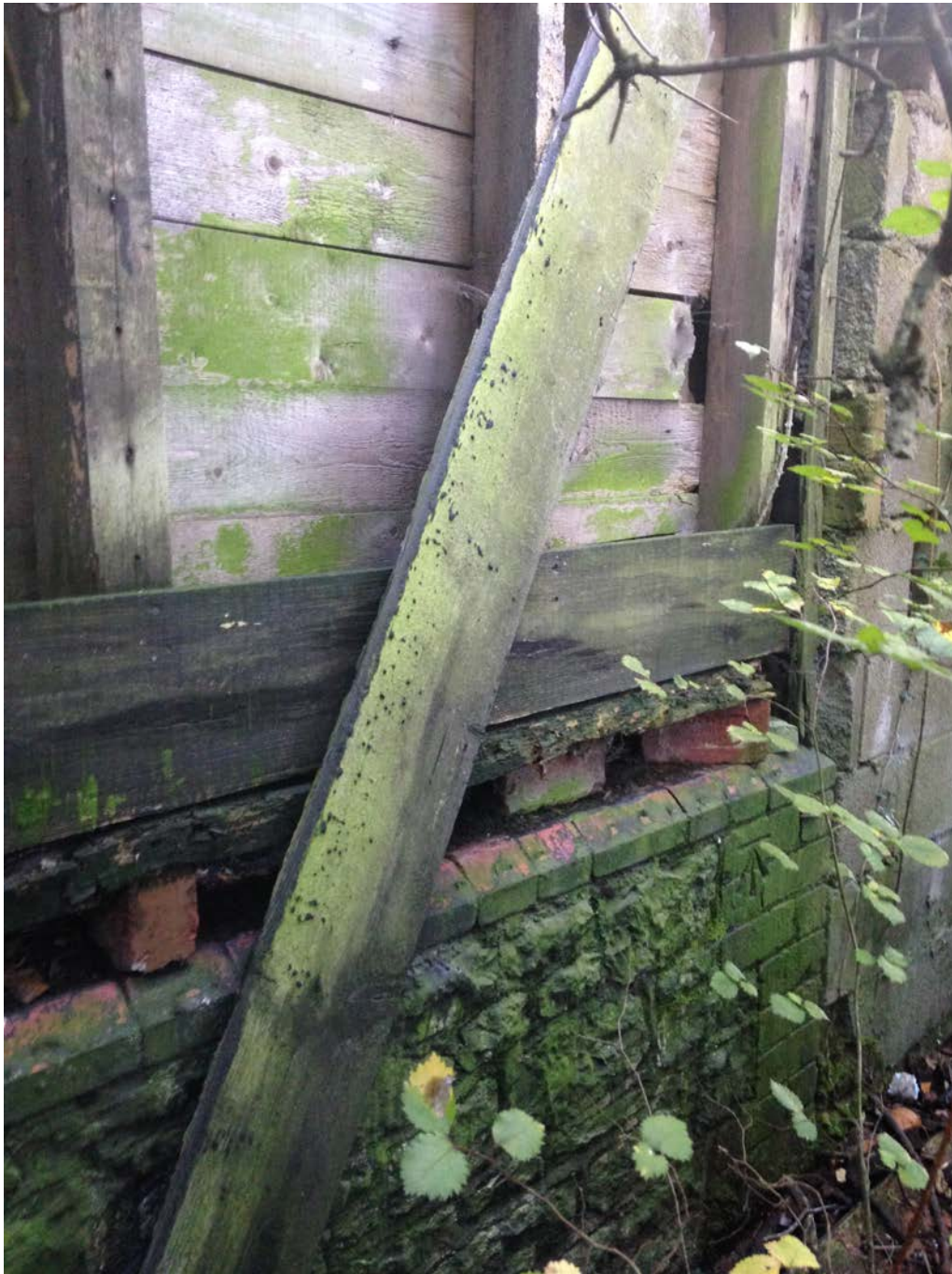
Image EDP 13: Depiction of the south west corner of the barn, here highlighting the use of basic modern materials to fill the gap between the timber sill beam and the stone and red brick dwarf wall characterising the outbuilding range
