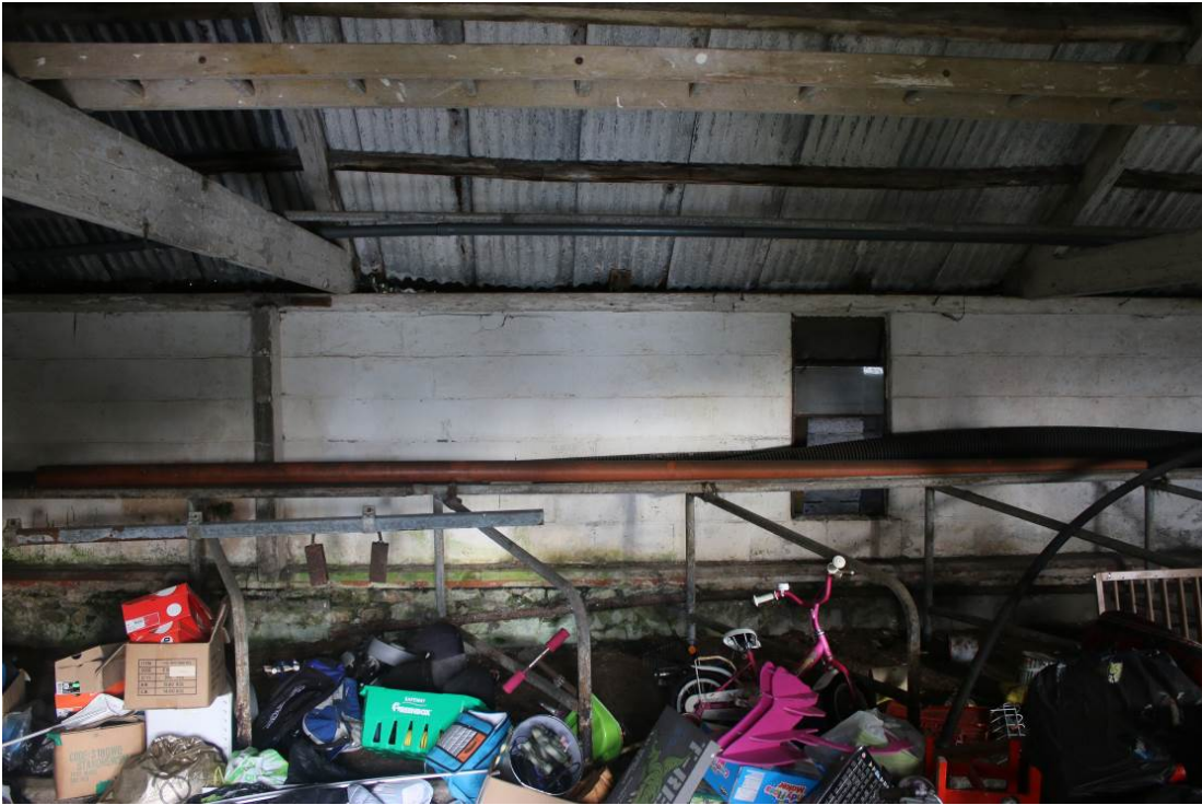
Image EDP 3: Photograph showing the continuation of the stone/red brick dwarf wall along the back wall of the northern range
