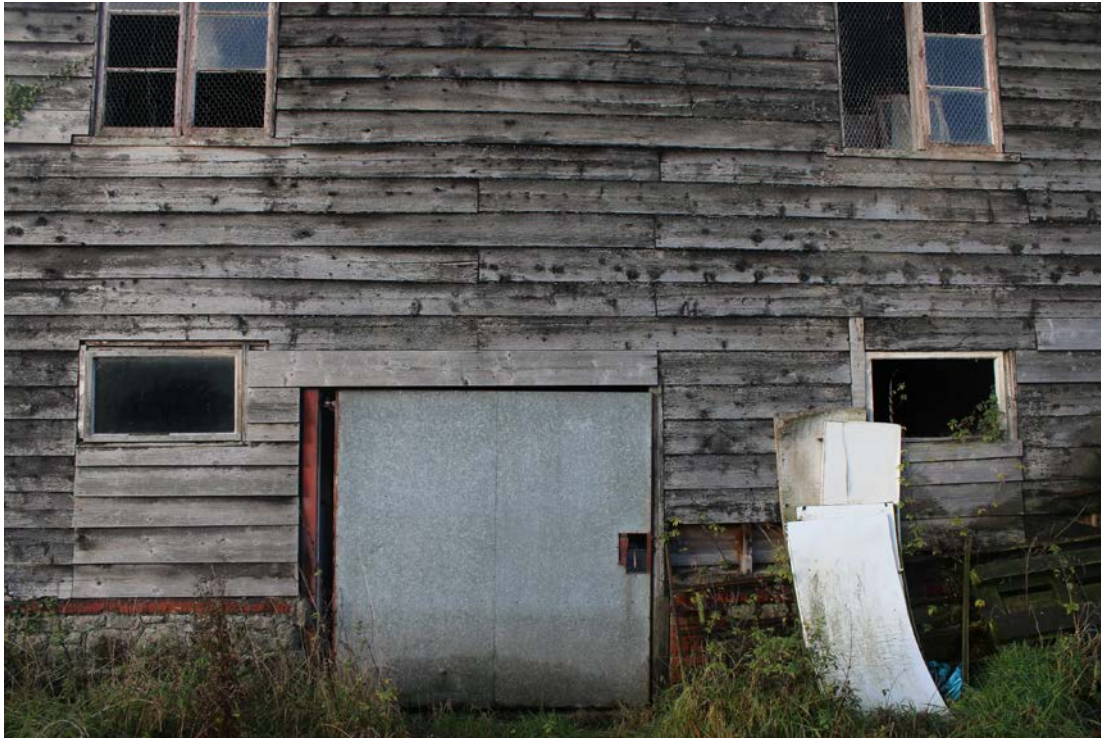
Image EDP 14: Close-up showing the relationship between the timber sill beam and the stone and red brick dwarf wall at the rear of the barn; clearly highlighting the use of basic materials
