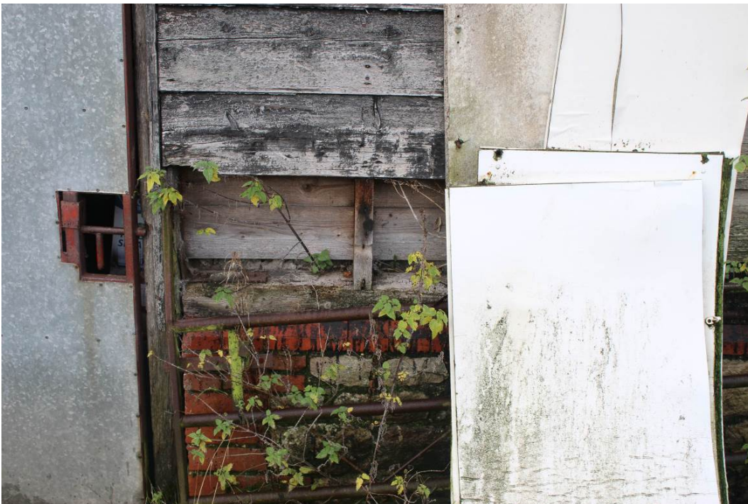
Image EDP 8: Close-up of the north side of the main door opening; here illustrating the neat brickwork which strongly suggests originality
