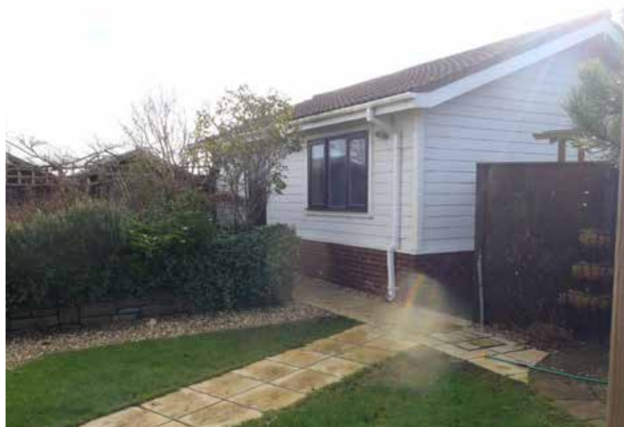
U-NORTH WEST VIEW OF DETACHED GARAGE
