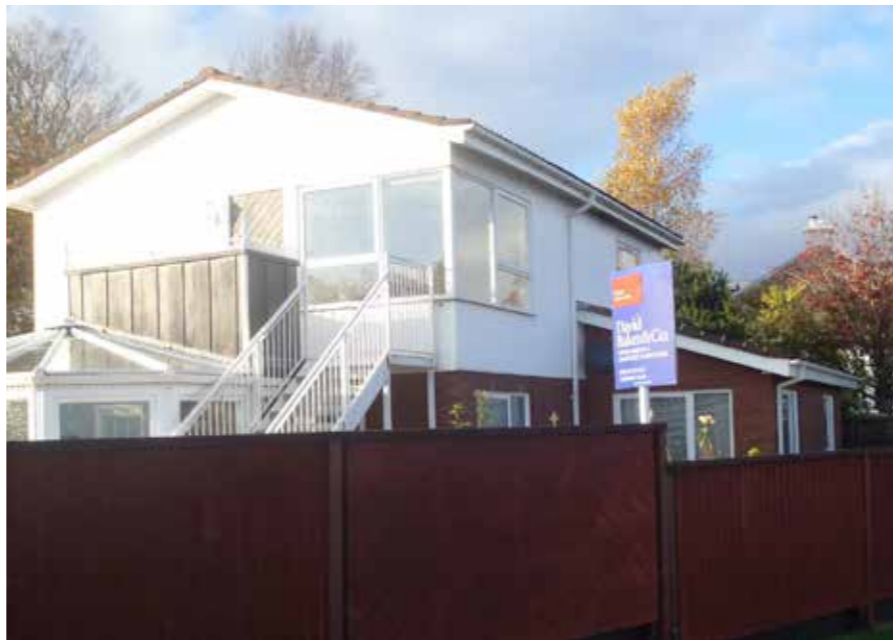
E-VIEW OF HOUSE (SOUTH & EAST ELEVATIONS) FROM CLIFF FOOTPATH
