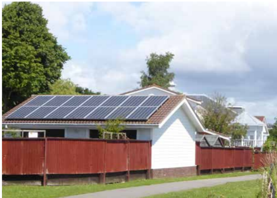
D-VIEW OF GARAGE (SOUTH & EAST ELEVATIONS) FROM CLIFF FOOTPATH
