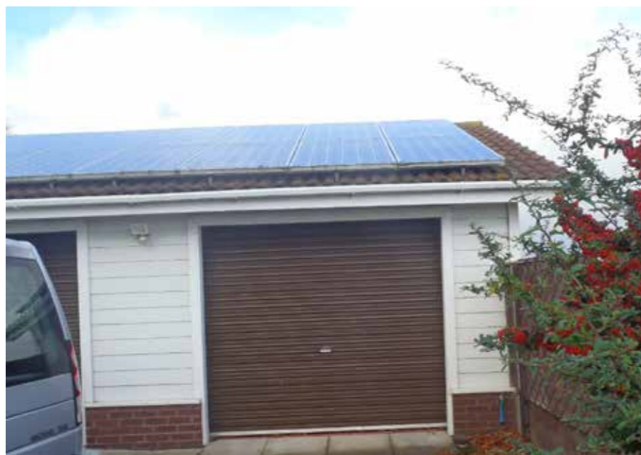
V-FRONT/SOUTH WEST ELEVATION OF GARAGE
