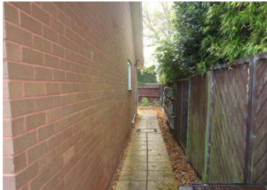
R-NORTH ELEVATION OF HOUSE FROM GREENHOUSE
