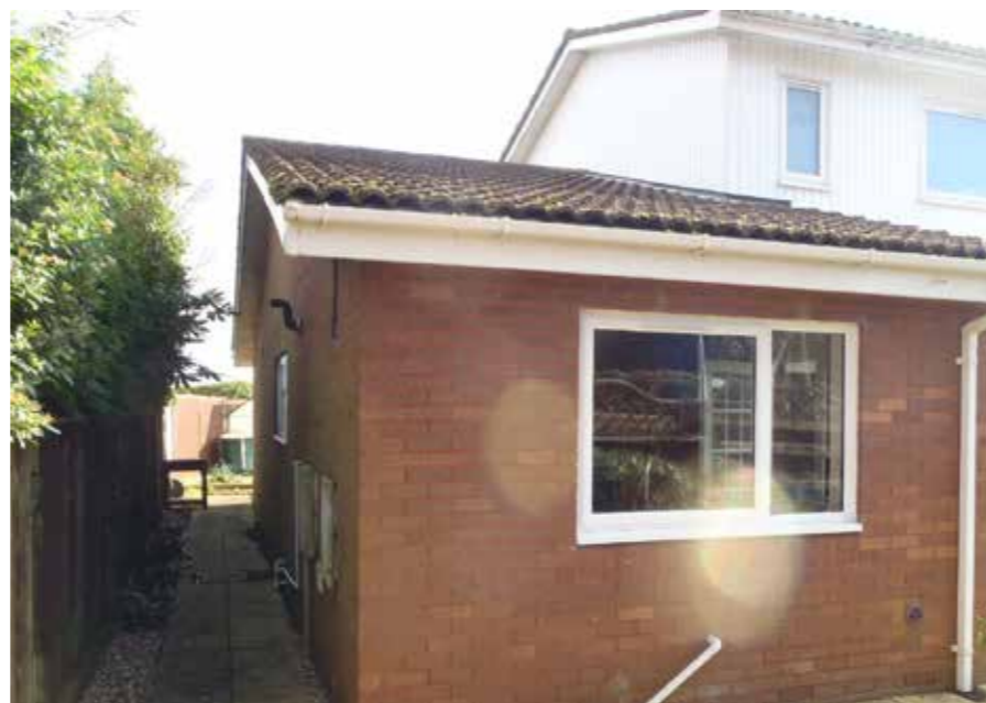
S-VIEW OF NORTH ELEVATION OF HOUSE TOWARDS GREEN HOUSE
