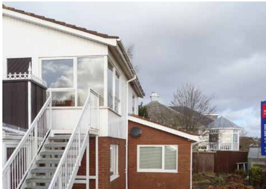
O-SOUTH VIEW OF HOUSE INCLUDING EXTERNAL STAIRS
