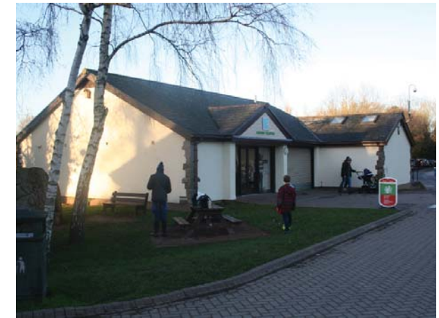
Existing Reception Building
