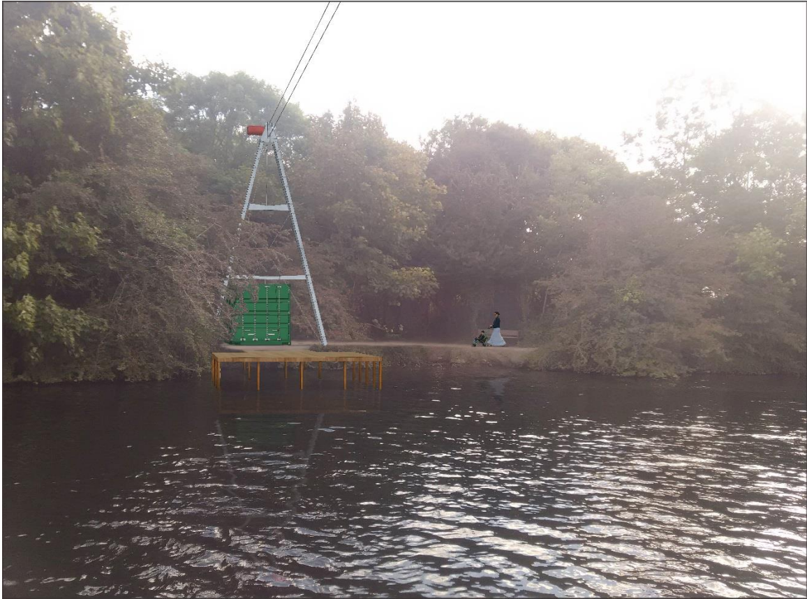
The start pontoon, system motor pylon and cable system storage container
