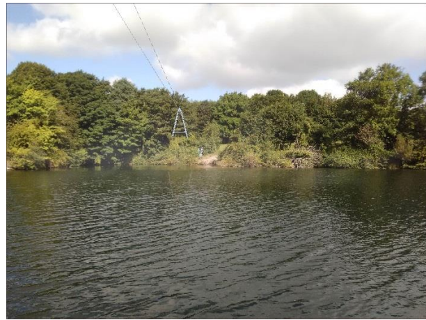
The supporting pylon on the Northern Bank
