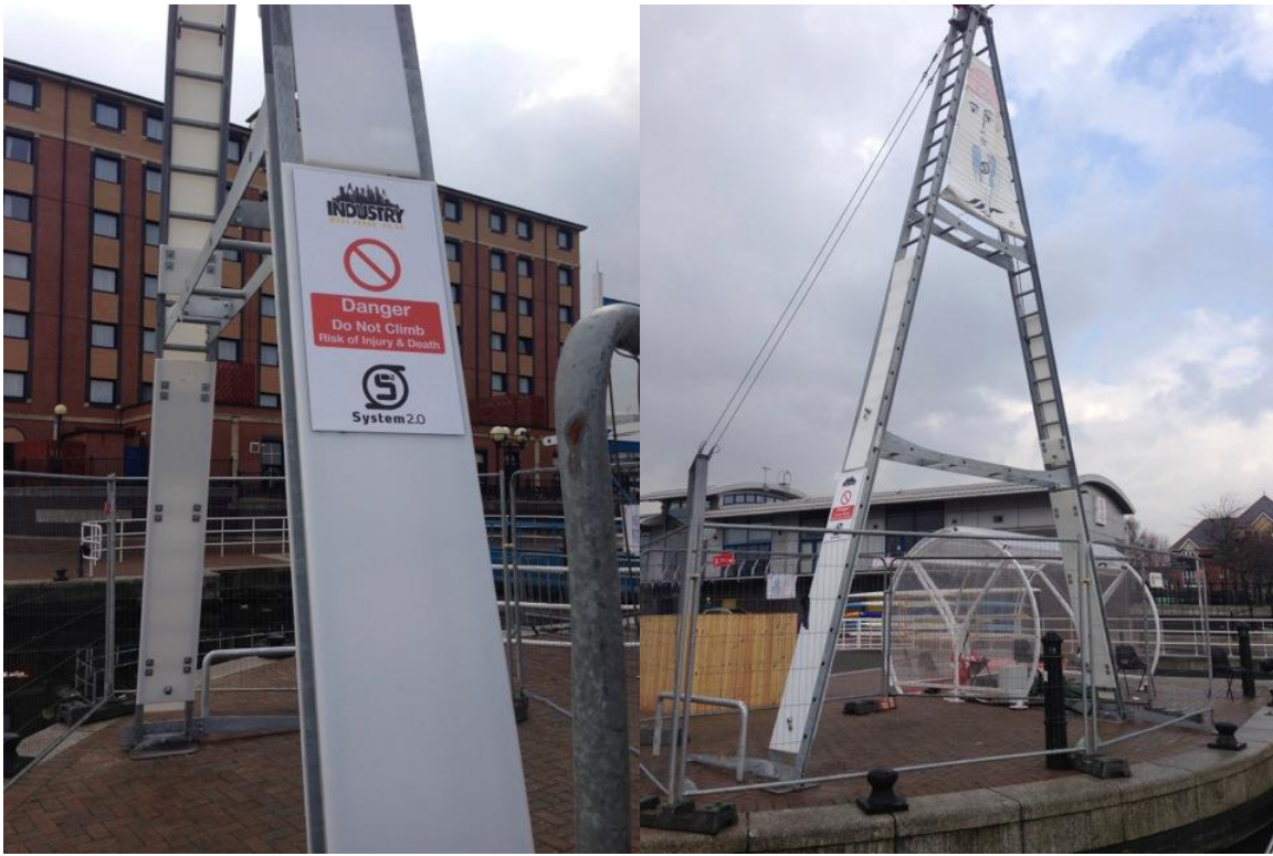
'No climb' panels installed at Salford Wake Park, UK
