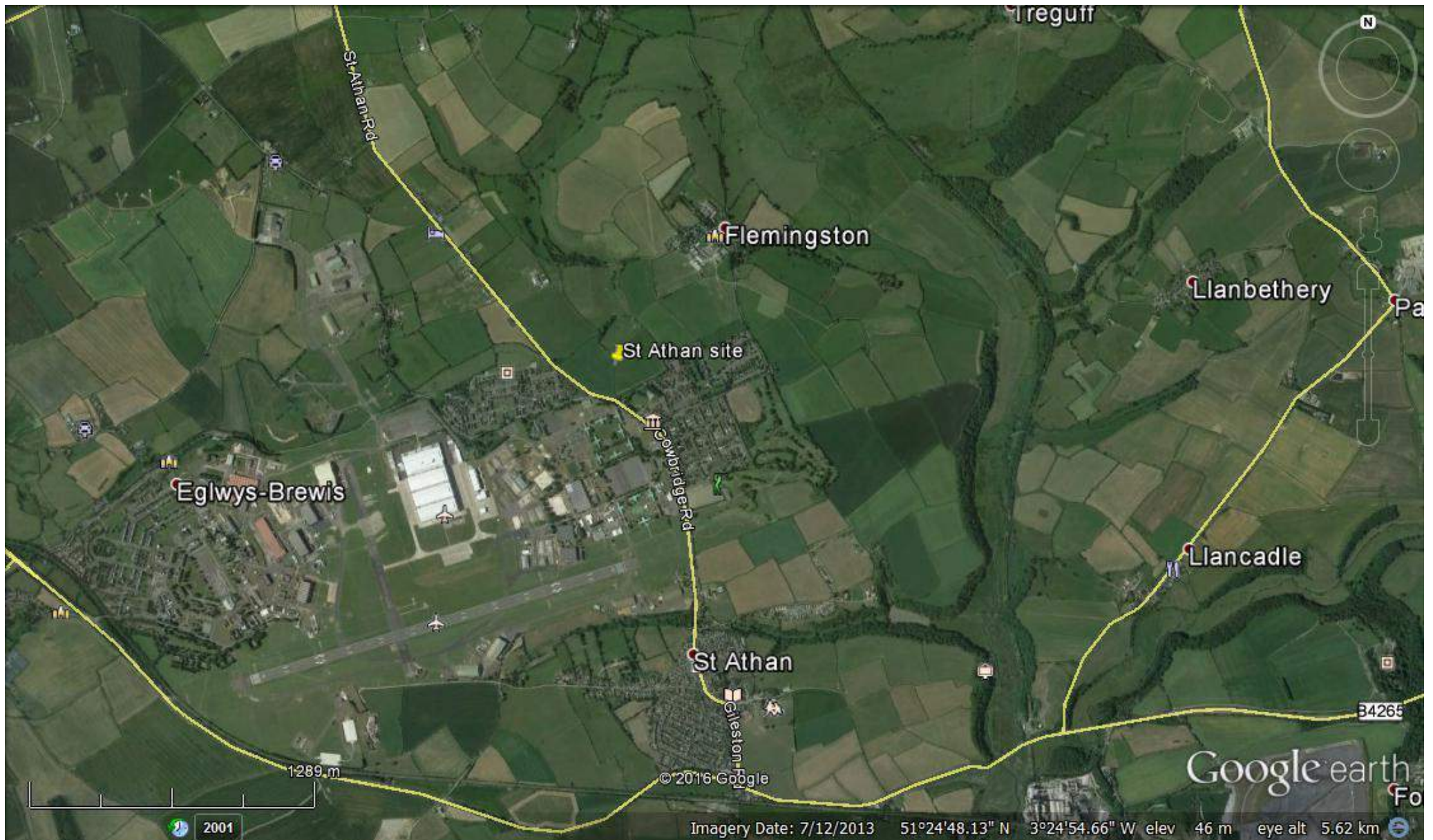
Aerial View showing location of St Athan survey area (Image Google Earth 2016)
