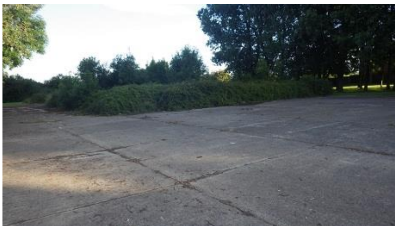
Plate 5 concrete hard standing
