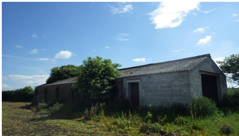
Plate 1 Building (1) barn with potential unrestricted access
