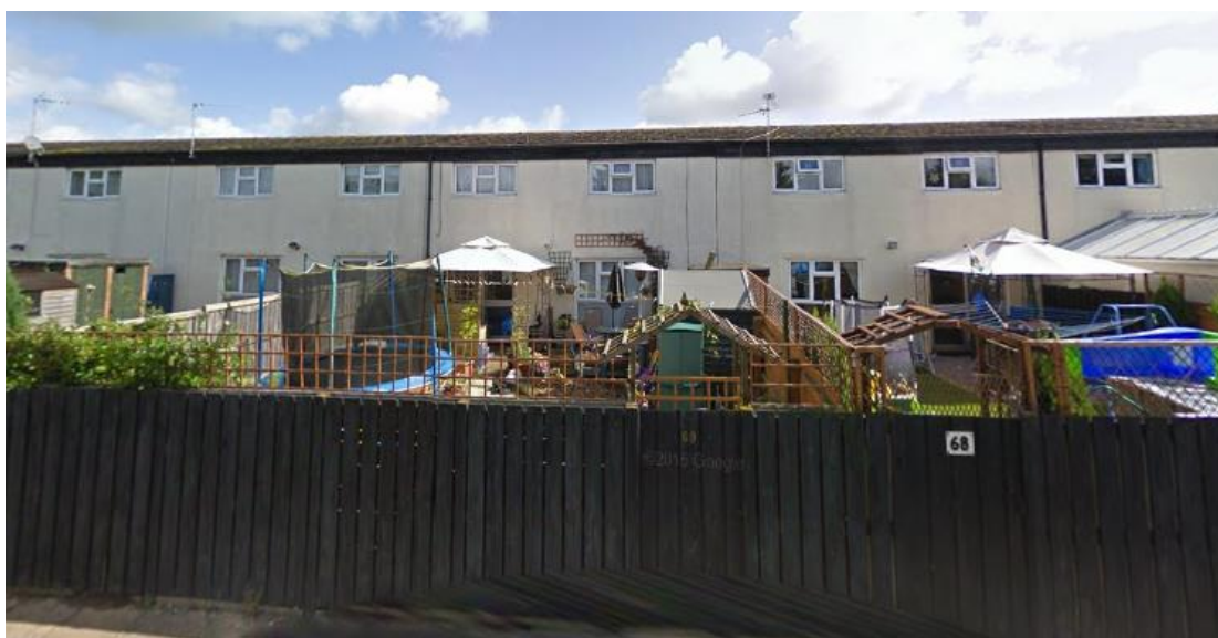
Existing dwellings located on Mallory Close
