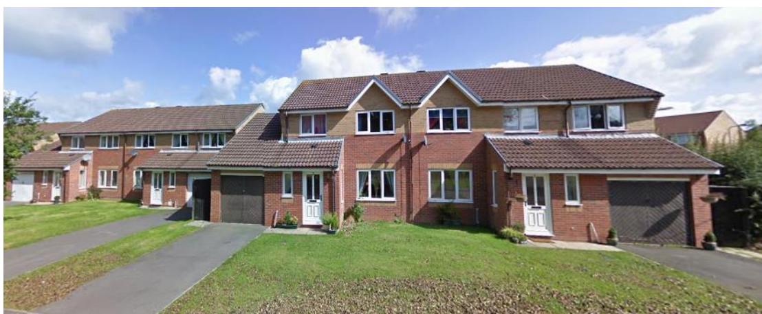
Existing dwellings located on Tintern Close
